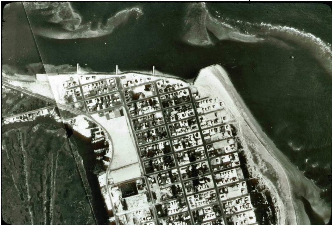
Figure 11. 1971 aerial photograph of Townsend's Inlet after construction of the 8 th Ave. jetty, the rock revetment and 3 short finger groins in the inlet. The main channel lies next to the revetment with vast shoals exposed at low tide immediately northeast of the channel. Note that the seaward parts of the shoal wrap around the inlet mouth and contributed large slugs of sand to the beach lying between the jetty and 17 th Street in Avalon. At this time there was a 465-foot wide vegetated dune system seaward of the end of 17 th Street before reaching the dry, high tide beach. Flood tidal currents and storm wave action moved sand over the jetty into the inlet where the ebb-tidal currents carried it back out to the shoals for eventual return to the north end beach. A stable cycle of sediment was in place. The jetty was also lower in elevation and shorter so that sand did move back into the inlet from Avalon generating a feed-back loop process. Deposits of sand washed over the jetty or around it were rapidly re-positioned by the ebb-tidal currents to the offshore bar and eventually back onto the Avalon ocean beach. The bar at the extreme lower right in the photograph is the point of attachment for sand moving landward from the offshore ebb-delta deposit.
