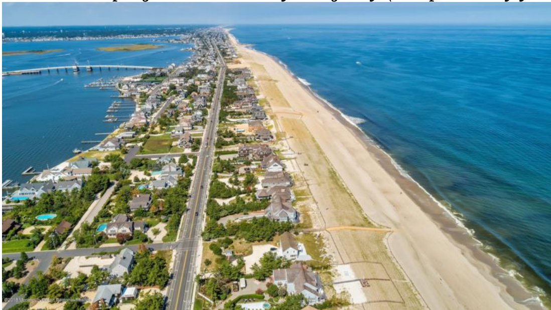
By 2019 the federal shore protection project was complete radically altering the Mantoloking oceanfront. The 22-foot elevation dune and the wider beach all provide massive storm protection and the steel wall is still present inside the dune.
