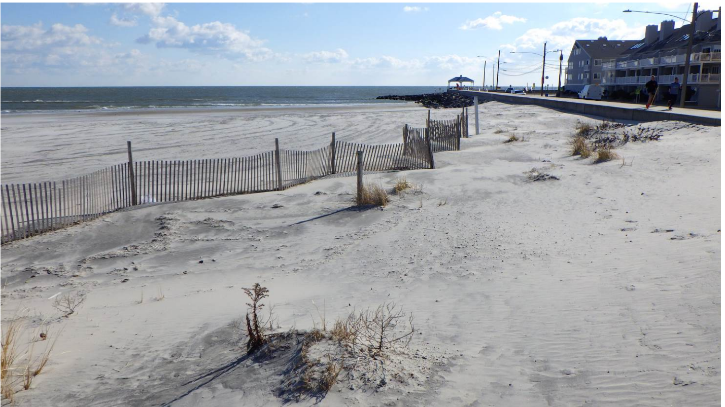
Figure 26. This view on January 22, 2021 shows a view to the southeast along the toe of the dunes. The bathing beach is substantial in width with a taper to zero width at the 2 nd Ave. and Kennedy Blvd. gazebo. The site stability is tied to loss from the oceanfront sand deposited each year derived from Wildwood City beaches. Flood tides act in concert with wave activity to move sand past the jetty into Hereford Inlet and it deposits along the inlet shoreline as an extended sand spit oriented into the inlet, along the City shoreline. Material initially deposits in the nearby offshore allowing ocean waves to move it landward adding to the beach eventually.
