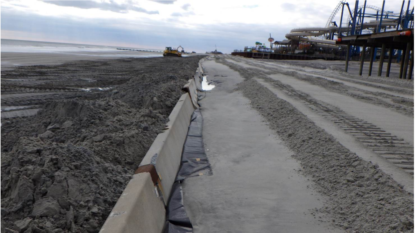
Figure 20. The January 27, 2021 view to the south looks across the front of the timber pier with the sand haul road in place to ease the trip past the pier at high tide. Morey's Surfside Pier can be seen in the distance further south with a wide, flat beach exposed at low tide.
