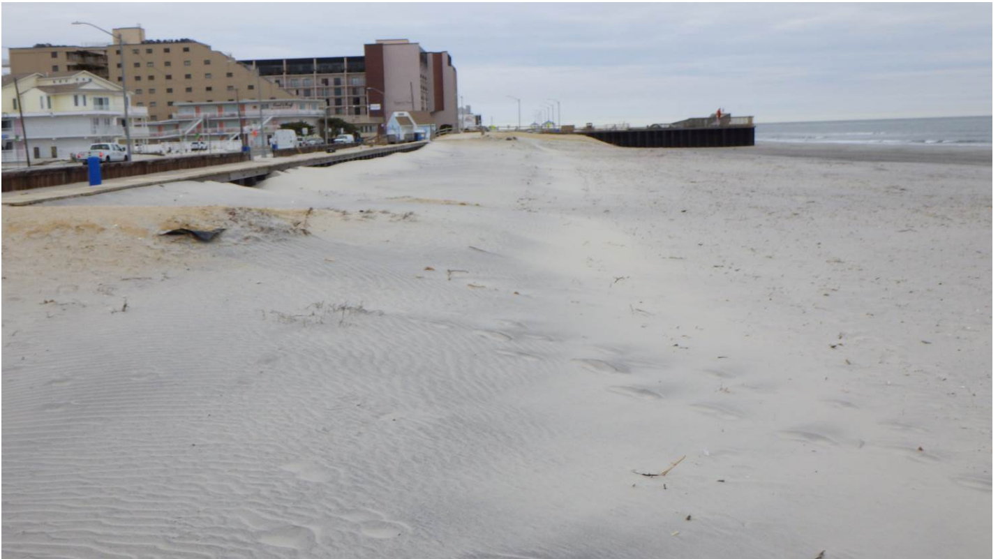
Figure 14. View to the north taken from the beach at 10 th Ave. on January 21, 2021 following loss of the dune constructed in 2009. The new steel bulkhead is partially buried in sand, but there is little added protection from the beach/dune system remaining.
