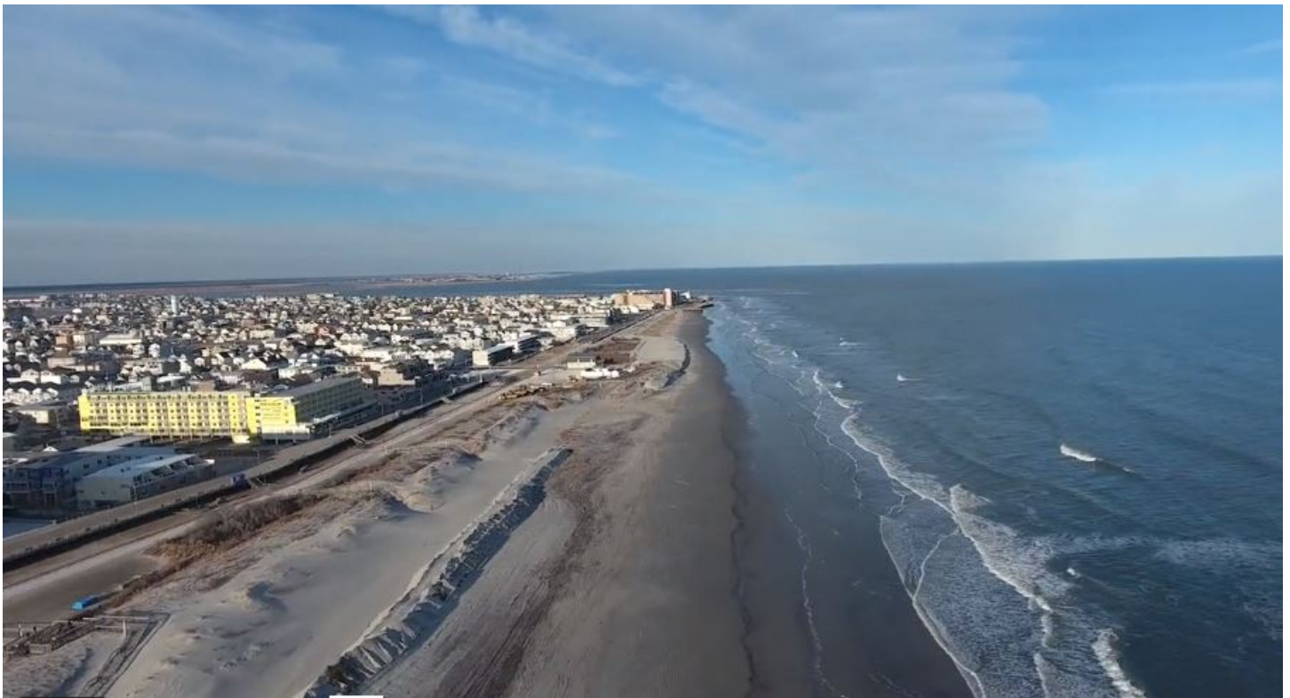
Figure 1. This Feb. 6, 2021 view looking north from a point just north of the first timber pier shows the extent of the damage. The beach is wet to the dune ridges and at the bulkhead/revetment north of 7 th Avenue.
