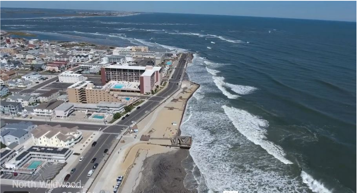
Figure 4. This Sept 22, 2020 view of the north end beach shows waves at the revetment and at the steel wall on a clear day with sizable surf coming in from the east, northeast.
