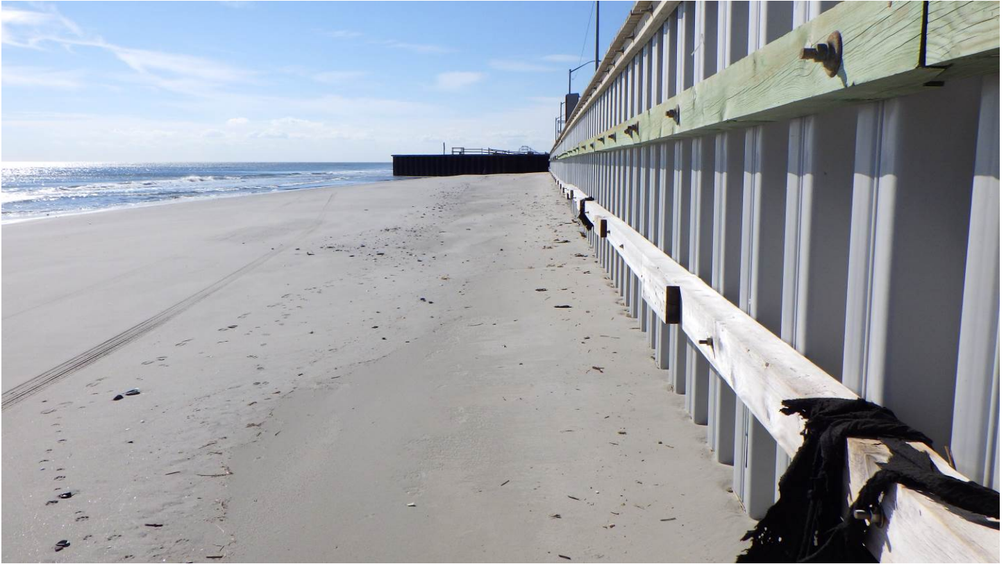
Figure 10. View to the south taken from directly in front of the new bulkhead that starts just south of the 3 rd Avenue gazebo on Jan. 22, 2021. The beach was wet to the bulkhead and only about 60 feet wide to the water at low tide. Waves reach the hard structures at any elevation of mid tide and higher. During the past summer there was a dry beach composed of Wildwood City sand transported north into the area.
