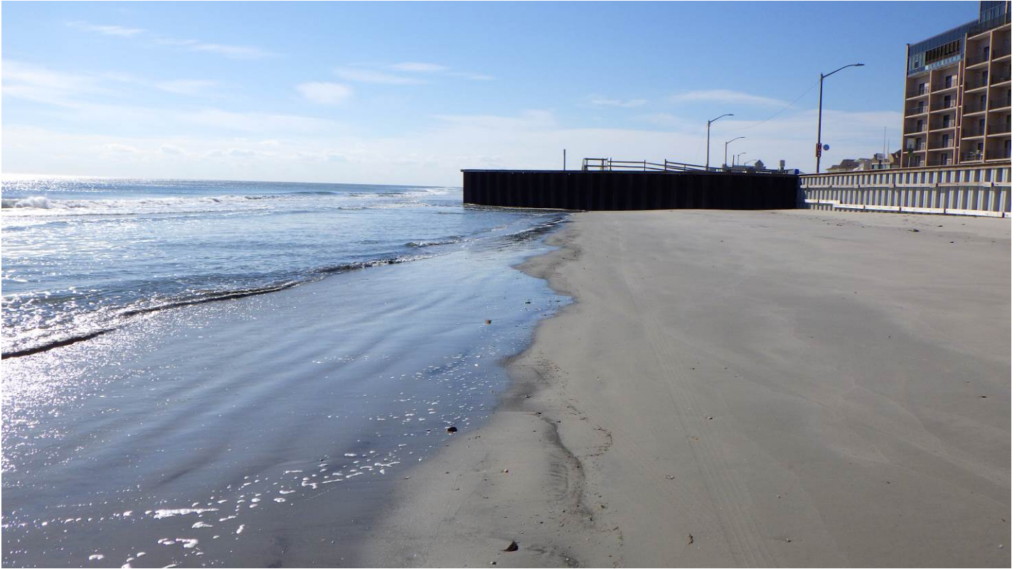
Figure 12. Site 06+00 is on the beach slightly north of where the new steel bulkhead extends seaward into the surf zone. The beach is a bit wider than at the 04+00 site, but high tide still reaches the bulkhead each time. The wave conditions on Jan 22, 2021 were extremely mild and the water was still at the bulkhead during the previous high water.
