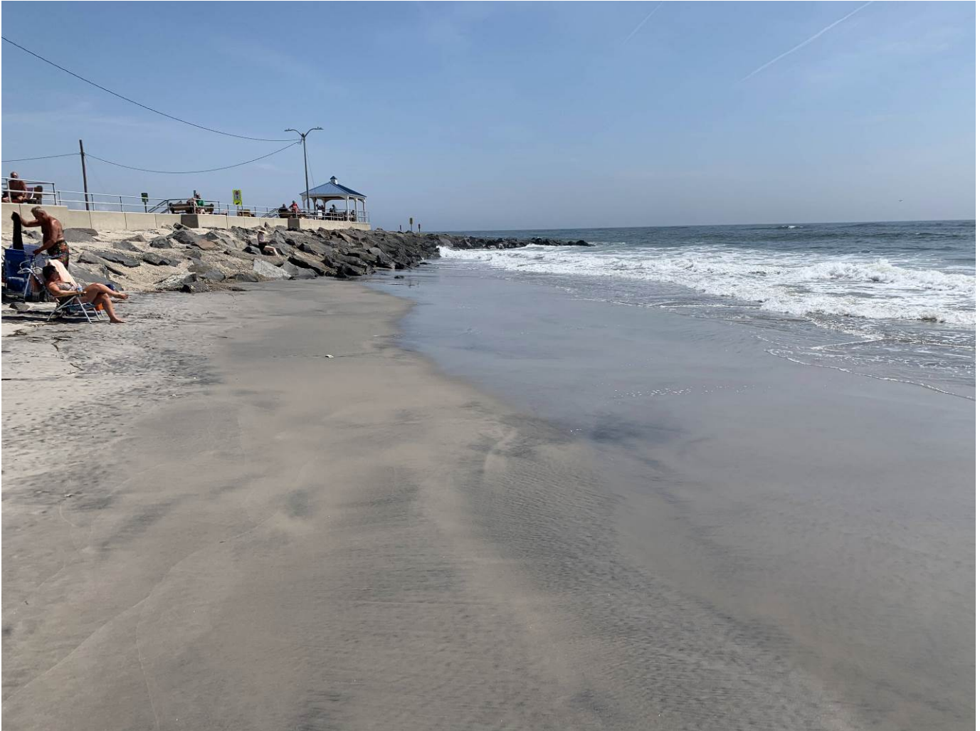
Figure 6. View to the north taken July 8, 2020 showing the inlet gazebo and inlet jetty beach. The photograph covers the northernmost 200 feet of beachfront following sand placement. In Jan. 2021 no wet sand was exposed even at low tide.
