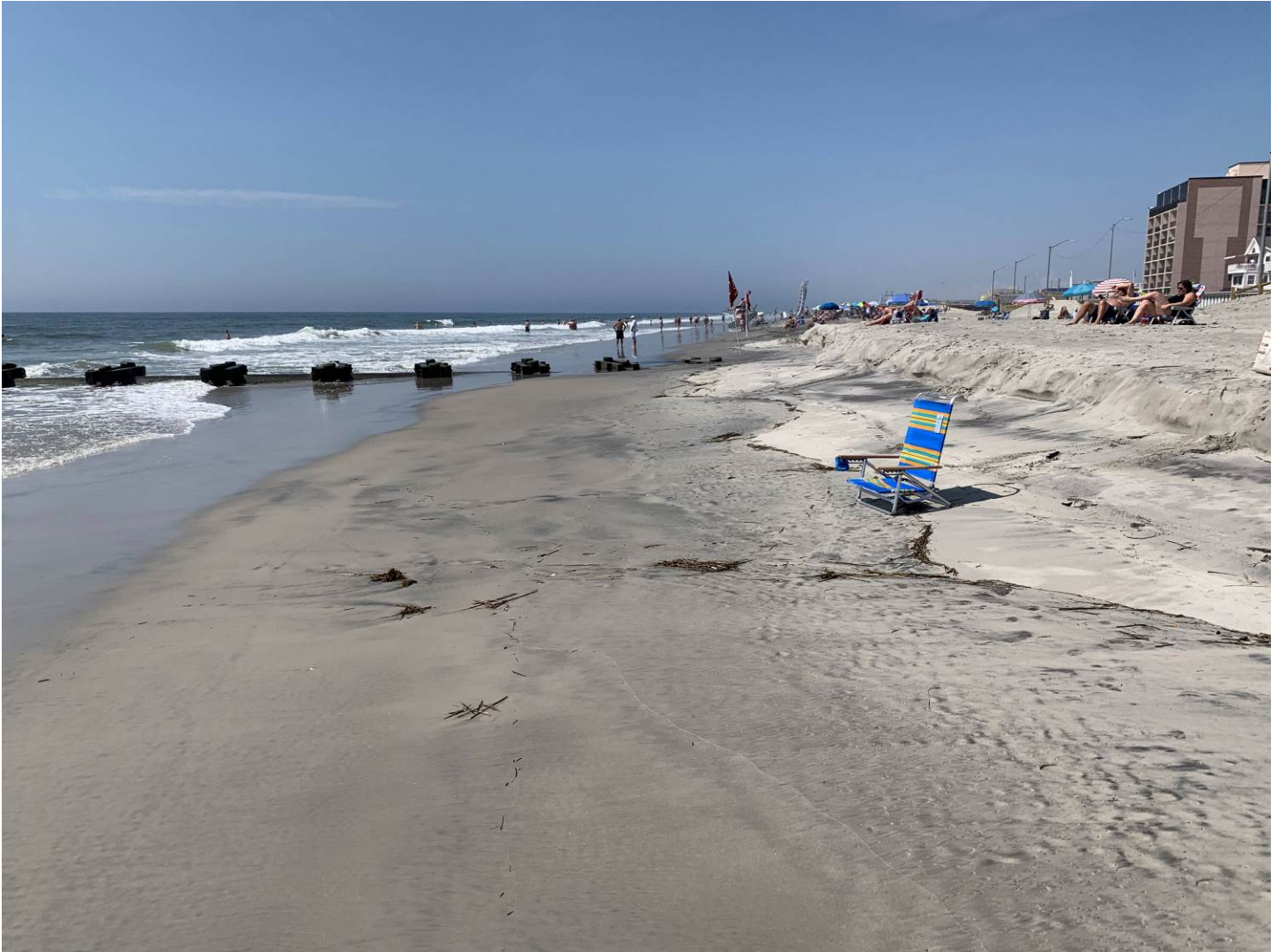
Figure 8. View to the south across site 02+00 and toward the stormwater pipeline showing the scarp cut into the back-passed sand volume on the beach as of July 8, 2020. There is sand offshore, but not in sufficient elevation or quantity to assist in providing any measure of adequate shore protection.
