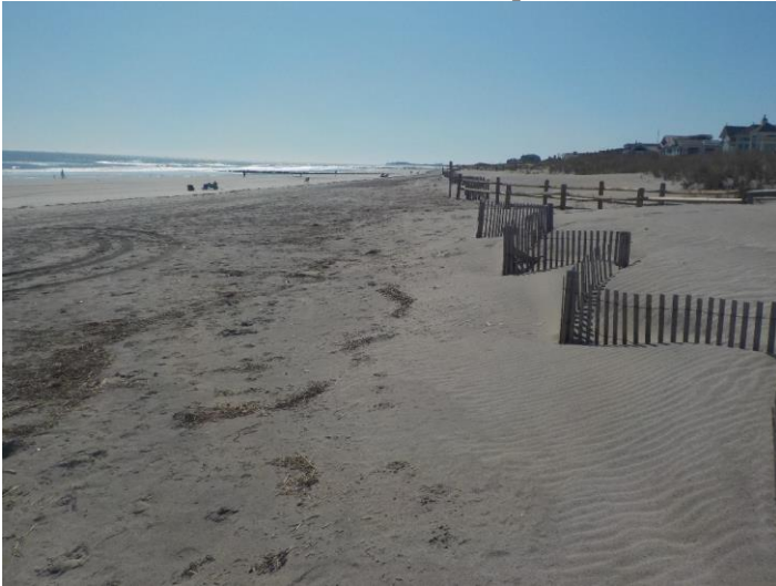
Photoplate 4a - Photo taken October 14, 2019 showing sand continuing to fill the 4-foot high snow fencing creating a new foredune. The beach width was sufficient to provide the supply.
