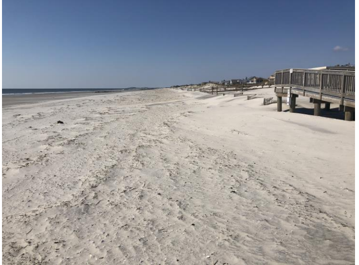
Photo 3b – The April 16, 2020 photo presents a wider dry beach with sand added to the nearly buried sand fencing at the toe of the seaward dune slope.
