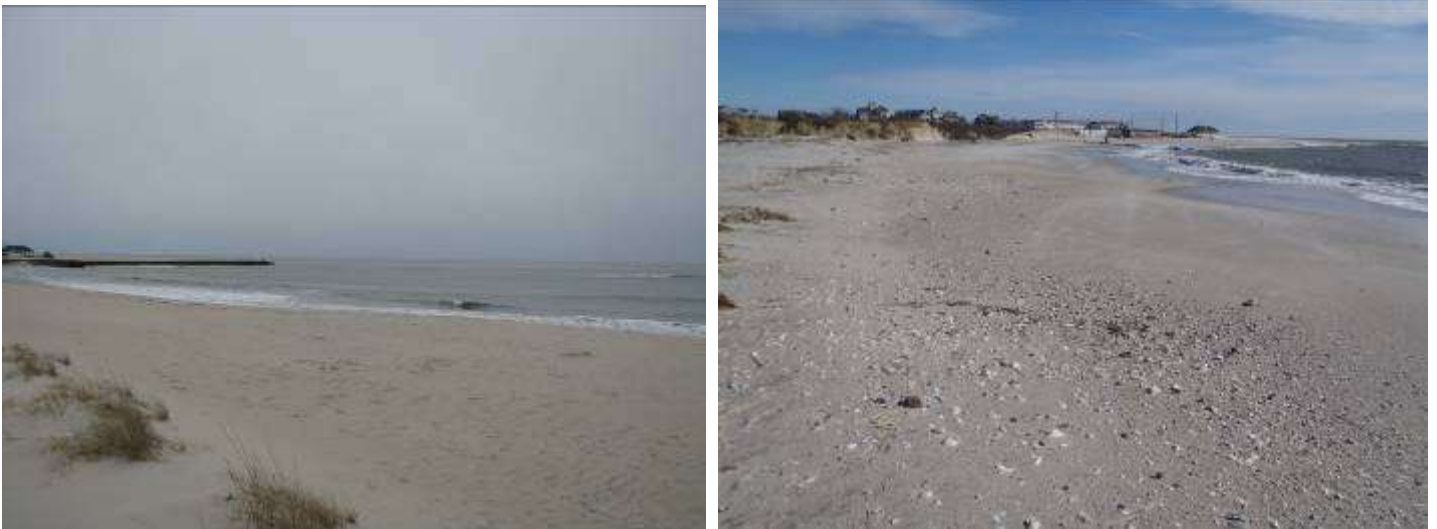
The left picture was taken March 5, 2012 looking toward the terminal groin in Cape May City. The left shot was done November 9 th showing the dune erosion and overwash into the newer dune development that has occurred over the past 22 years since the initial beach restoration took place in Cape May City in 1990.
