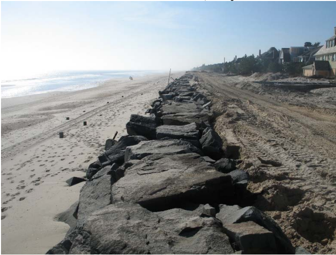
The community of Bay Head experienced wide-scale overwash during H. Sandy stripping away the low dunes and exposing the 5,500-foot rock revetment that was constructed after the 1962 northeast storm (left photo taken November 12, 2012). On the right, (September 3, 2013) sand recovered from the overwash deposits inland was returned to the beach to cover the rocks once again.
