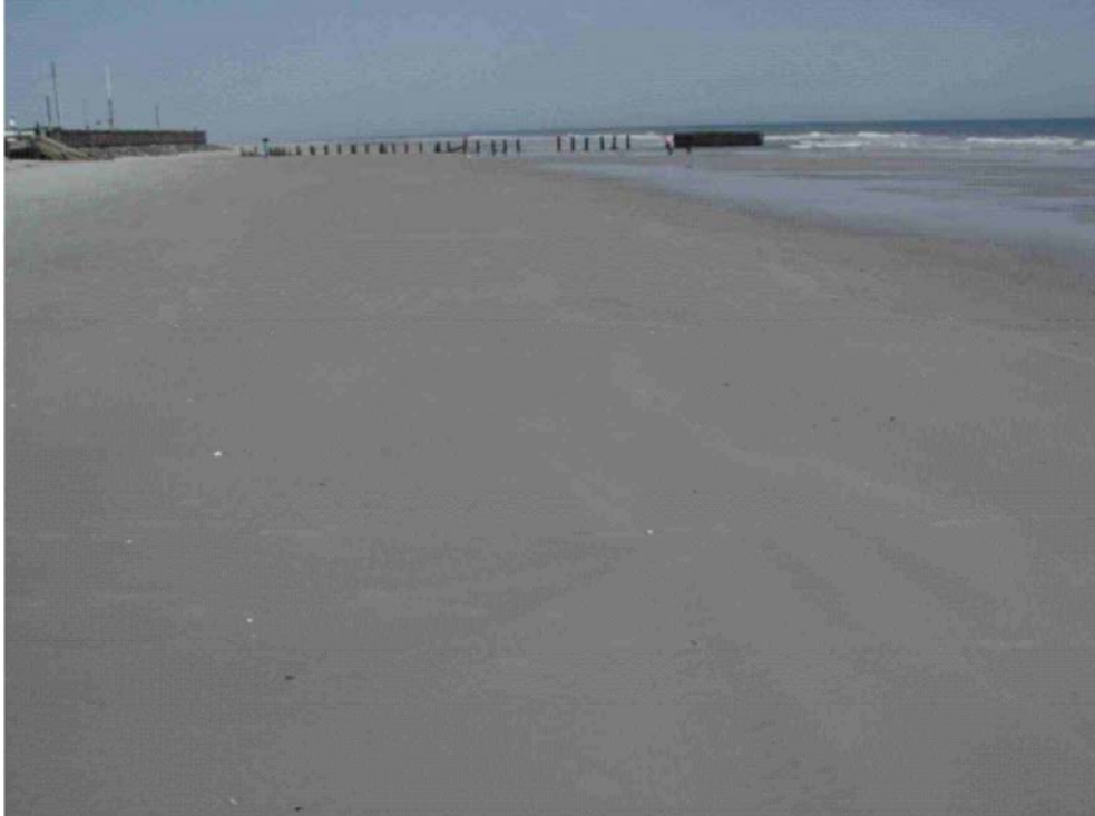
Photoplate 5a. While not an NJBPN profile site, this location is situated about 2000 feet north of site #133 in the zone of worst erosion. This shot was taken October 12, 2005 just prior to a northeast storm event that made this situation worse.
