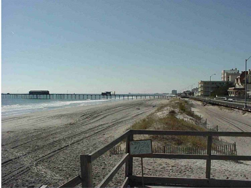
Photoplate 6a. A view of the Ventnor City beach from October 20, 2000 showing the limited width and elevation to the dune system prior to the ACOE Federal beach restoration project completed in 2002.
