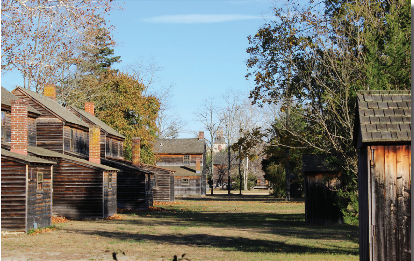
WORKERS HOUSES & MANSION, Batsto Village, Burlington County, 2014.
