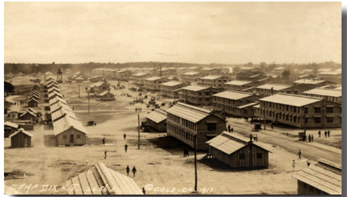
Camp Dix under construction, 1917
