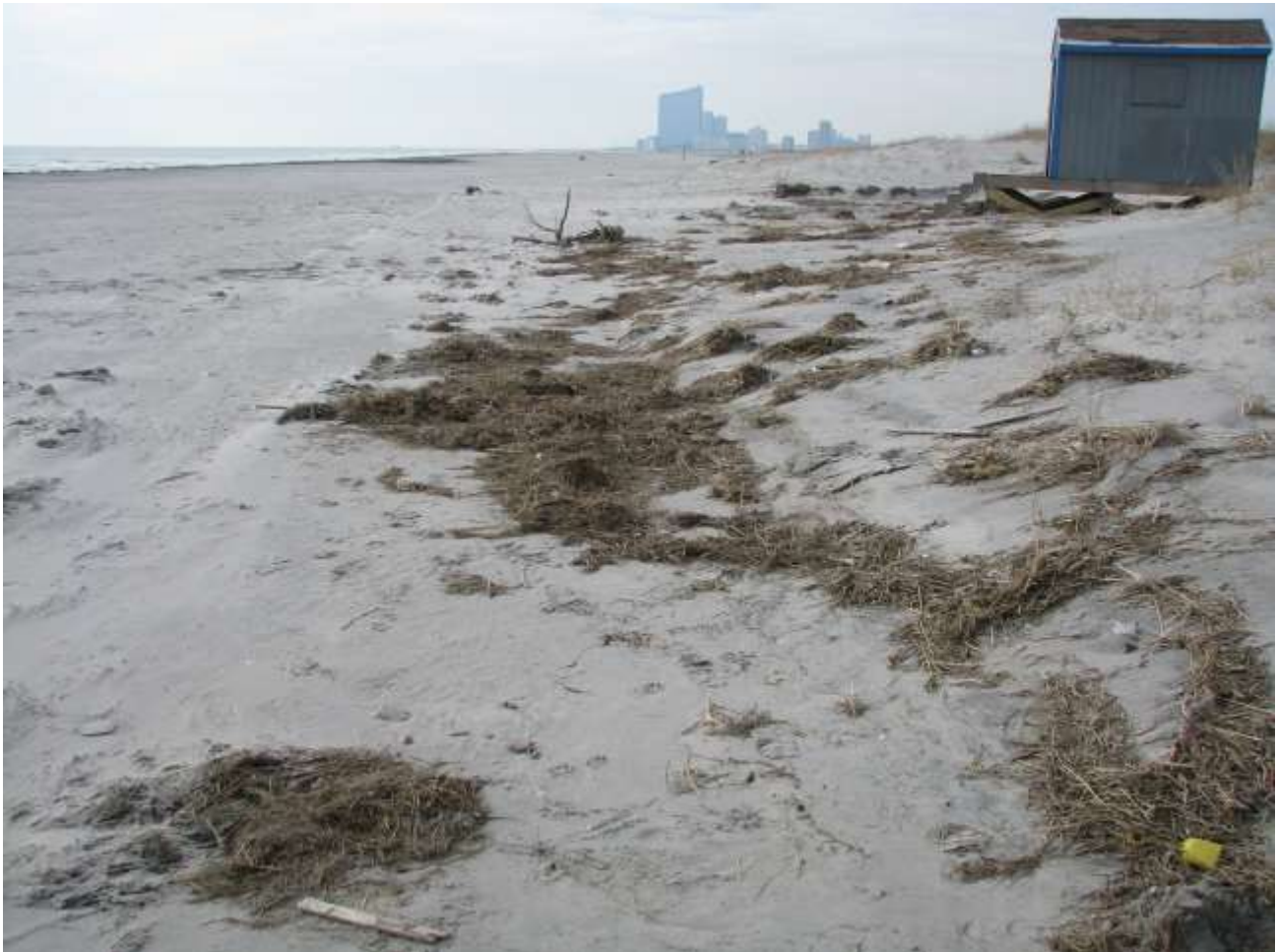
Figure 7c taken January 29, 2016, again looking south from the same location following winter storm Jonas. The thick debris wrack line is evidence that wave storm run up reached the seaward dune toe during Jonas. However, the wider beach berm did absorb most of the wave energy preventing any significant erosion along the dune toe in this region. The beach berm is slightly narrower following the storm but still wide enough to provide significant storm protection during future events.
