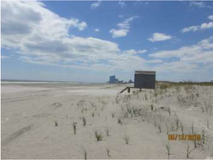
Figure 7a photo was taken looking south on May 13, 2015. Two years following Sandy natural aeolian accumulation of sand along the seaward dune slope fully restored and enhanced the seaward slope and toe. Grasses have colonized to the seaward toe.
