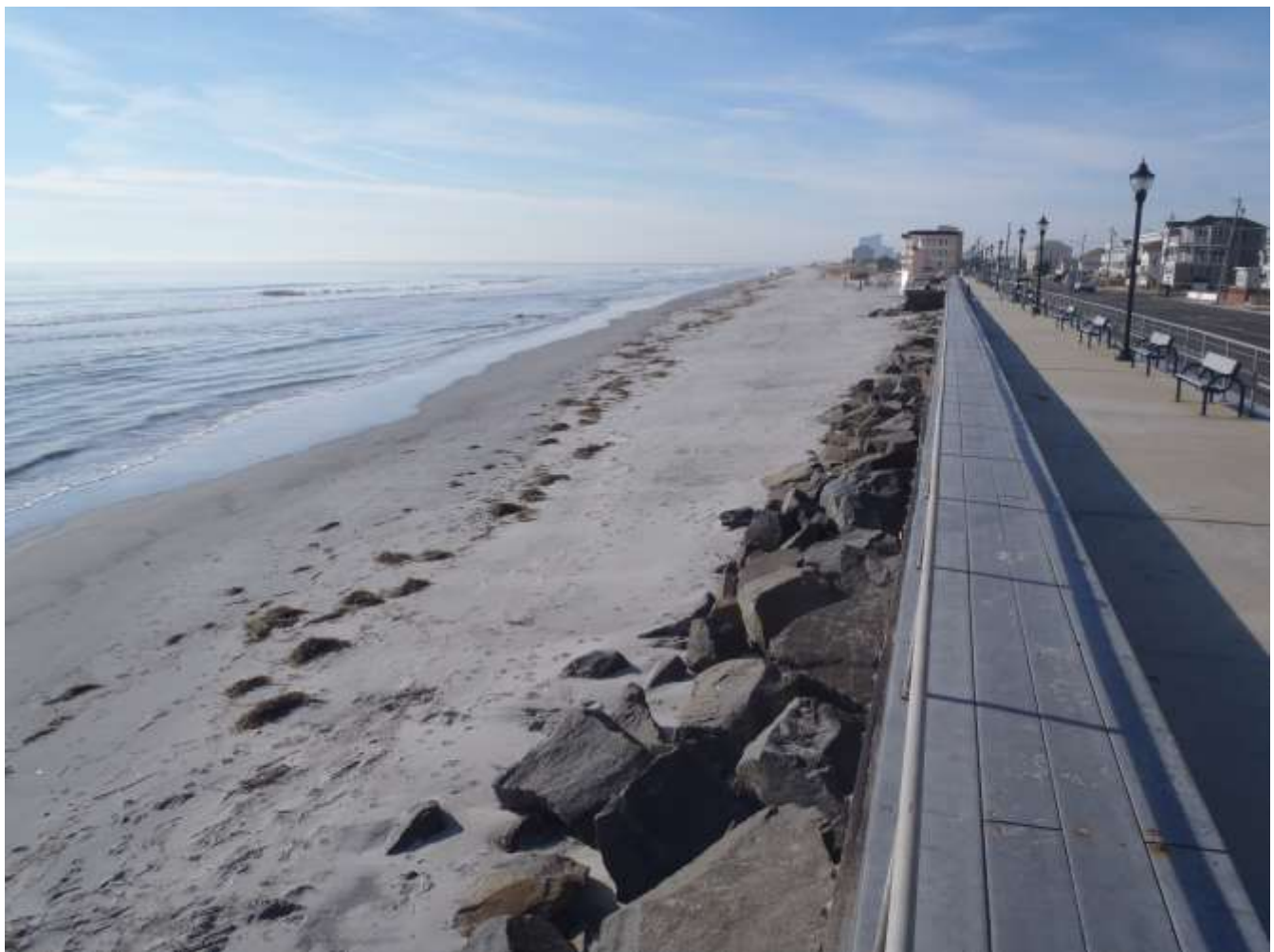
Figure 3c taken on January 27, 2016 this photo was taken from the same location following winter storm Jonas, a severe nor'easter. Photo shows a rapid deterioration of the beach conditions since October 2015 and exposure of the rock revetment. The orientation of the natural shoreline converges with the street end revetment and promenade in this location. Once the shoreline has retreated to the rocks, erosion rates accelerate from wave refraction off the hard structure resulting in a chronic erosional hotspot.
