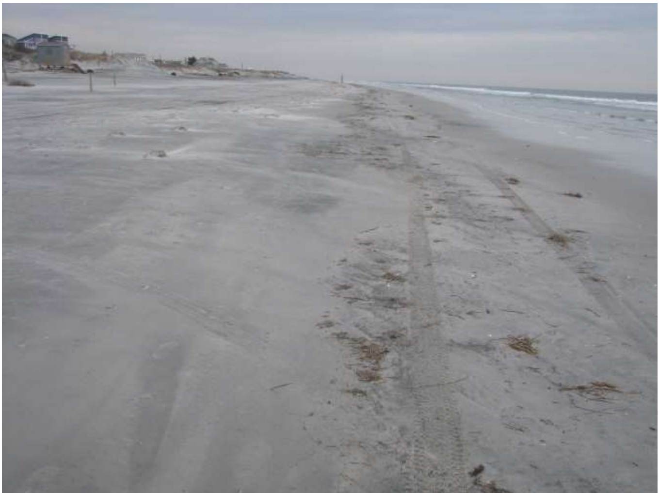
Figure 6c photo was taken looking north on January 29, 2016 following Jonas. Beach width and elevation have been further reduced but a sufficient wide beach berm remains to provide shore protection for the dune in the vent of future storm events.
