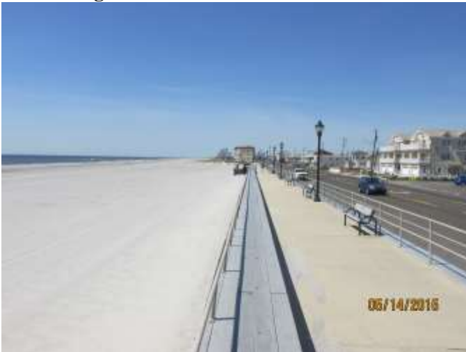
Figure 3a taken on May 14, 2015 the restored beach template remained relatively stable since completion of the 2013 USACE project. The mild 2014-2015 winter season were absent of severe storms allowing the wide beach berm to persist through to spring of 2015.
