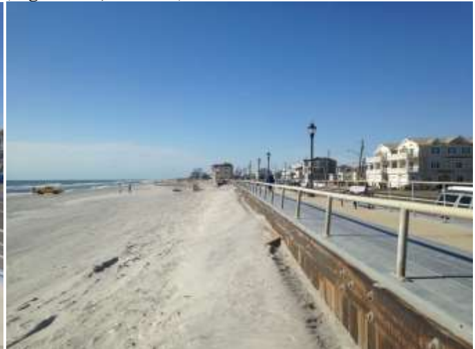
Figure 3b photo above was taken October 16, 2015 from a similar location. The wide beach berm still present in spring 2015 has been flattened by storm wave runup that nearly reached the revetment two weeks prior during the early October nor'easter.
