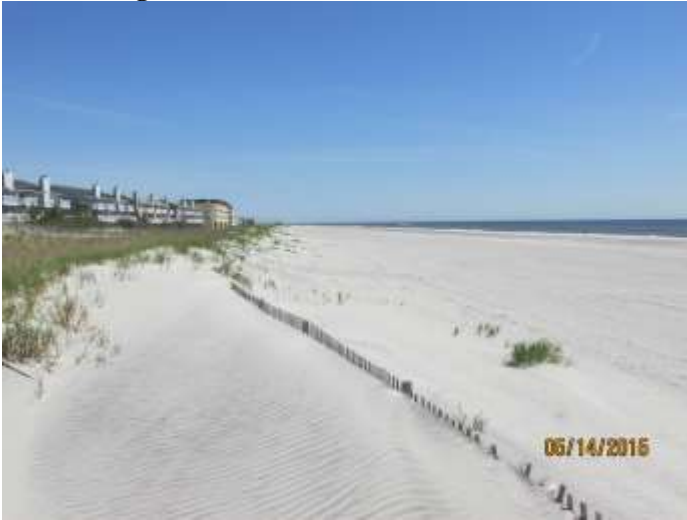
Figure 4a photo was taken looking north on May 14, 2015. This beach was fully restored to the design template two years prior. A new foredune has developed burying the installed fence, early colonizing plants have begun to propagate.
