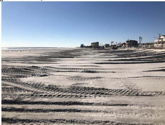
**Figure 3b** taken October 30, 2018 shows the completed work on the beach by the USACE. The bulldozer pushed up material to the top of the bulkhead while the rocks were covered during sand slurry placement.
