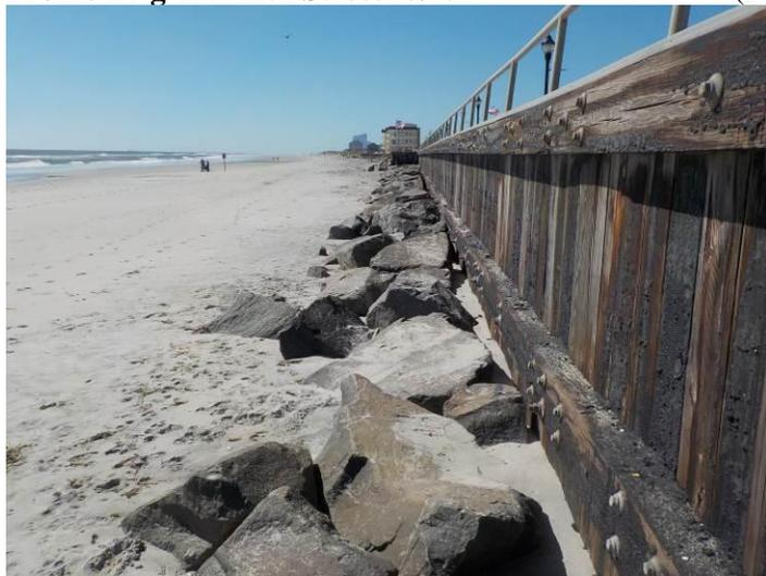
**Figure 3a** taken October 2, 2017 following the summer beach accretion. A small berm had developed filling in around the rocks leaving a narrow dry beach in place.
