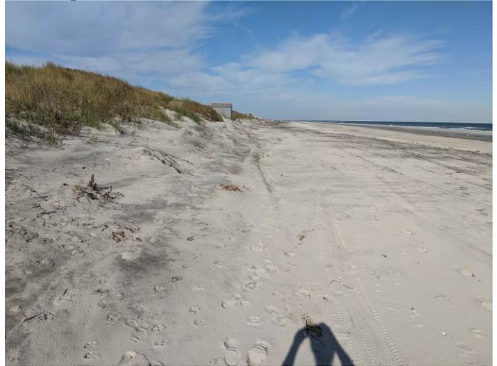
**Figure 5b photo taken October 15, 2019 looking north along the seaward toe of the dunes showing the sand added to the dune slope and a wide, stable beach seaward.**
