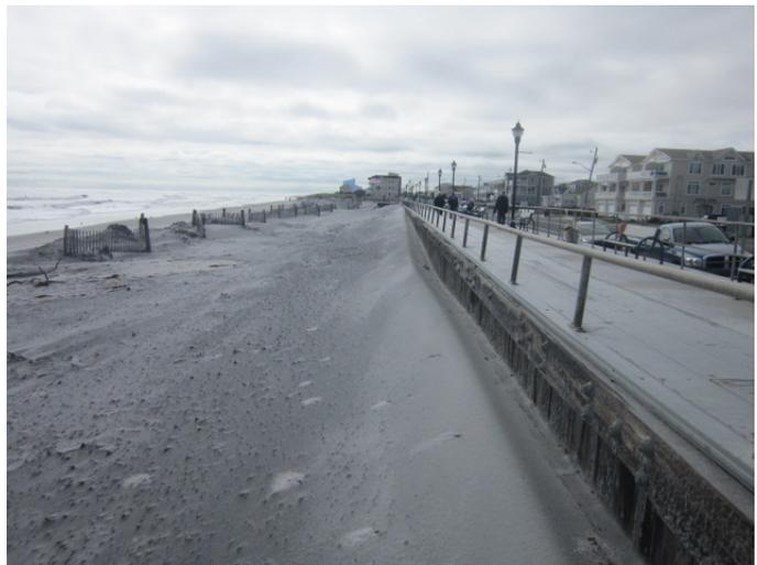
**Figure 3b taken October 13, 2020 with the sand fence at the swash limit and only about 25 feet of berm left to the promenade wall. The rocks remain buried at this moment.**
