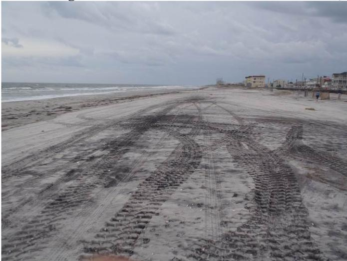
**Figure 3a taken October 16, 2019 is a view from the beach berm crest looking south showing that the beach has retained most of the sand placed in 2018 by the USACE.**
