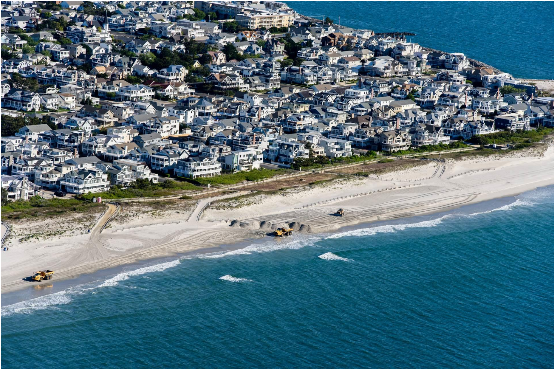
Figure 3a. May 13, 2021 aerial view of the Avalon back-passing depositional zone between 12 th and 15 th Streets where the truck loads are dropped off and then graded into the desired beach template. Erosion continues its work between 11 th and 17 th Streets so beach utility depends on regular episodes of sand addition to keep the resource functional as both storm protection and a recreational space.
