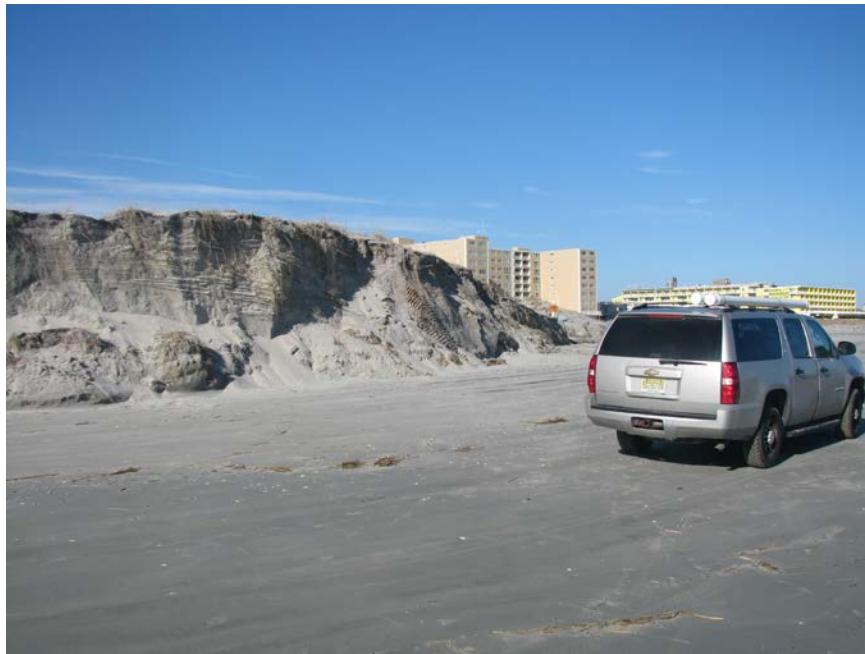
Figure 26. A close up view of the dune looking to the north from the beach located near 22 nd Avenue on January 27, 2016. Jonas caused severe erosion to the dune where a large scarp can be seen.
