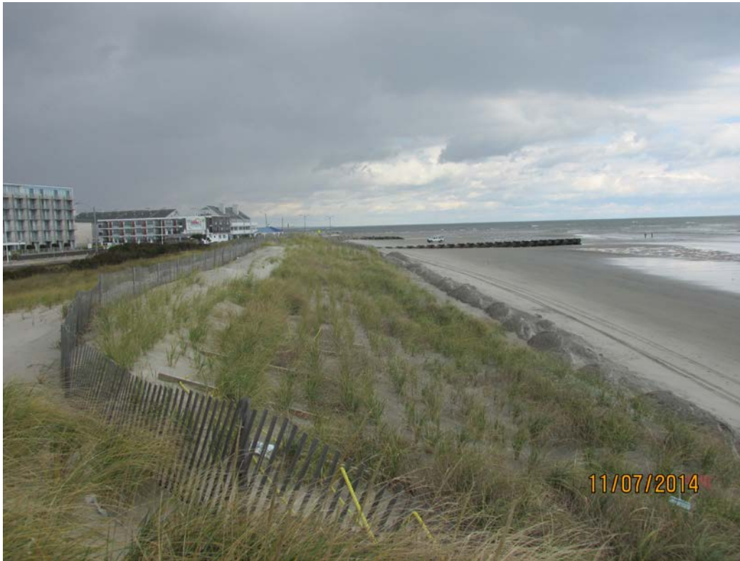
Figure 5. View from 5th Avenue looking north taken on November 7, 2014 displaying trucked-in piles of sand at the seaward dune toe. Nearshore bar gains had taken place since April 2014 while the dune and beachface remained stable. From November 2013 to November 2014 the shoreline remained virtually unchanged while below datum gains of 8.81 yds 3 /ft. were recorded.
