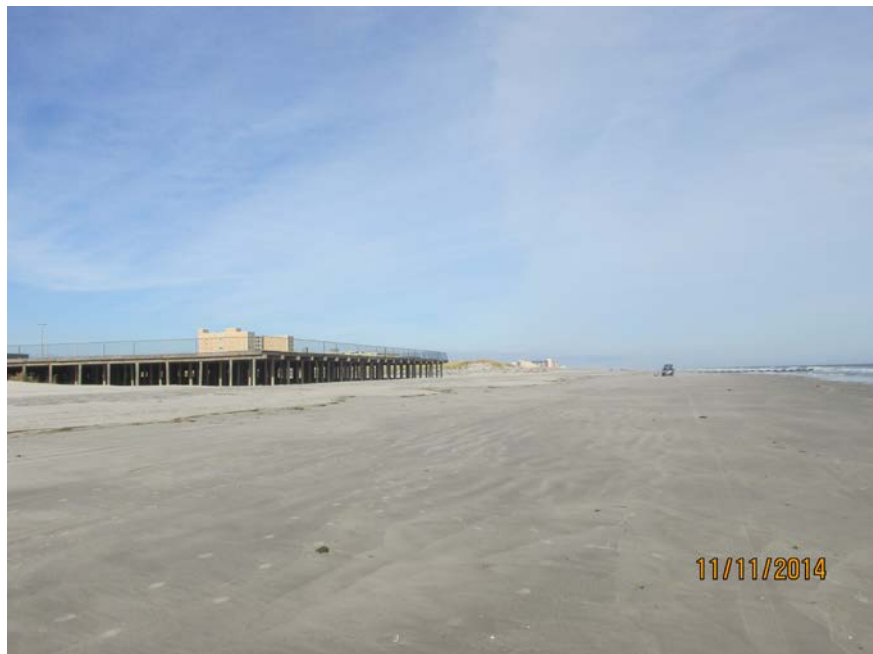
Figure 19. View to the north taken on November 11, 2014 near 25 th Avenue showing the configuration of the beachface. The two surveys conducted in the spring and fall 2015 revealed approximately a 2-foot lower elevation in this region than that pictured above.
