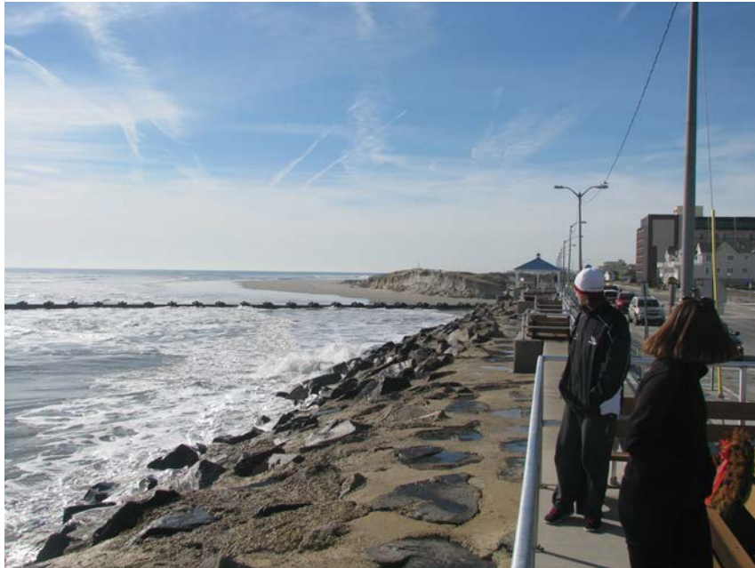
Figure 24. A close up view of the exposed seawall looking to the south at 2 nd Avenue on January 25, 2016. Winter Storm Jonas eroded sand in this area completely exposing the wall at virtually all stages of the tide cycle.
