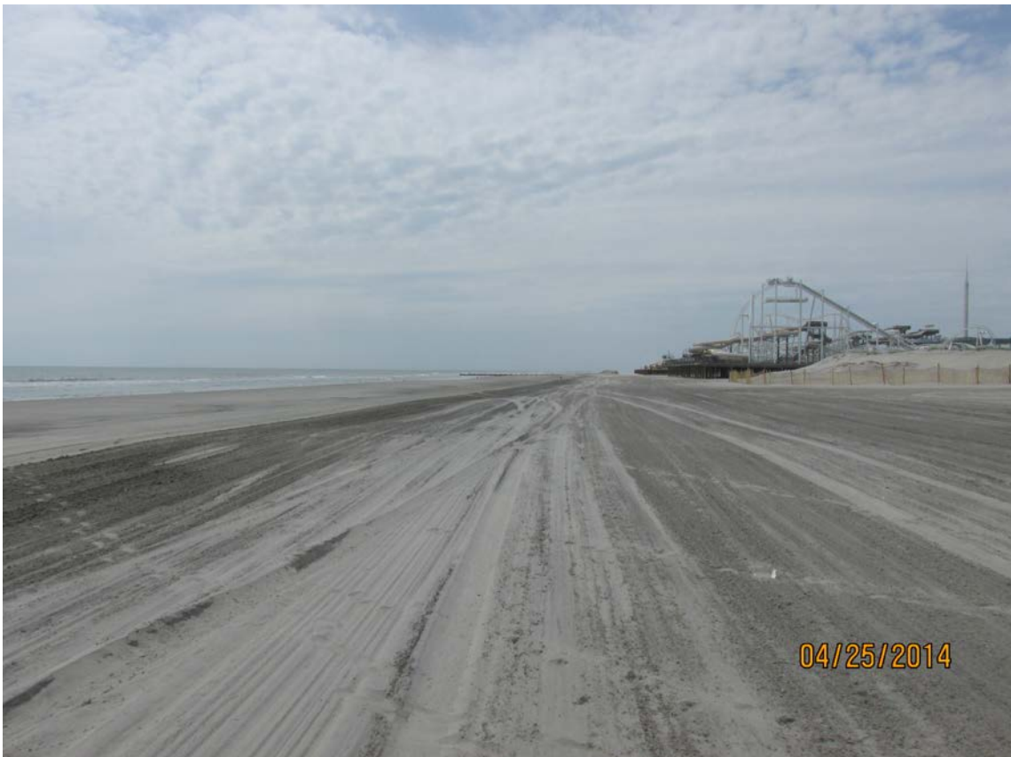
Figure 16. View to the south from the beach located near 22 nd Avenue on April 25, 2014. This location did not receive any sand directly during the 2013 beachfill. Erosional processes prevailed in 2014 overall but the wider beach width seaward of the dune allowed for Aeolian sand to be deposited at the dunecrest.
