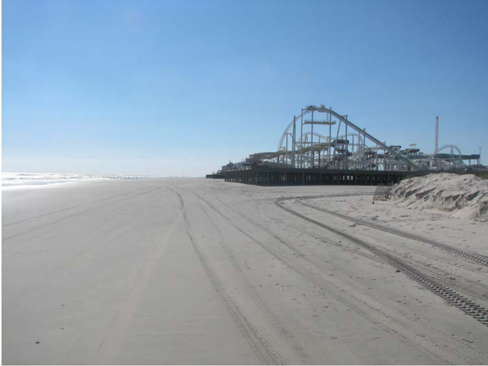
Figure 20. A close up view of the dune looking to the south from the berm located near 23 rd Avenue on October 30, 2015. The low elevation of the beach is clearly displayed resulting in a small scarp to the seaward dune toe.
