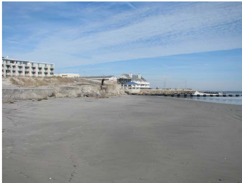
Figure 25. View to the north following Jonas taken at 5 th Avenue on January 25, 2016. The storm caused severe erosion to the beach and dune system creating the large scarp seen in the dune and the remainder of the sand from the Beach Creek dredge material pile.
