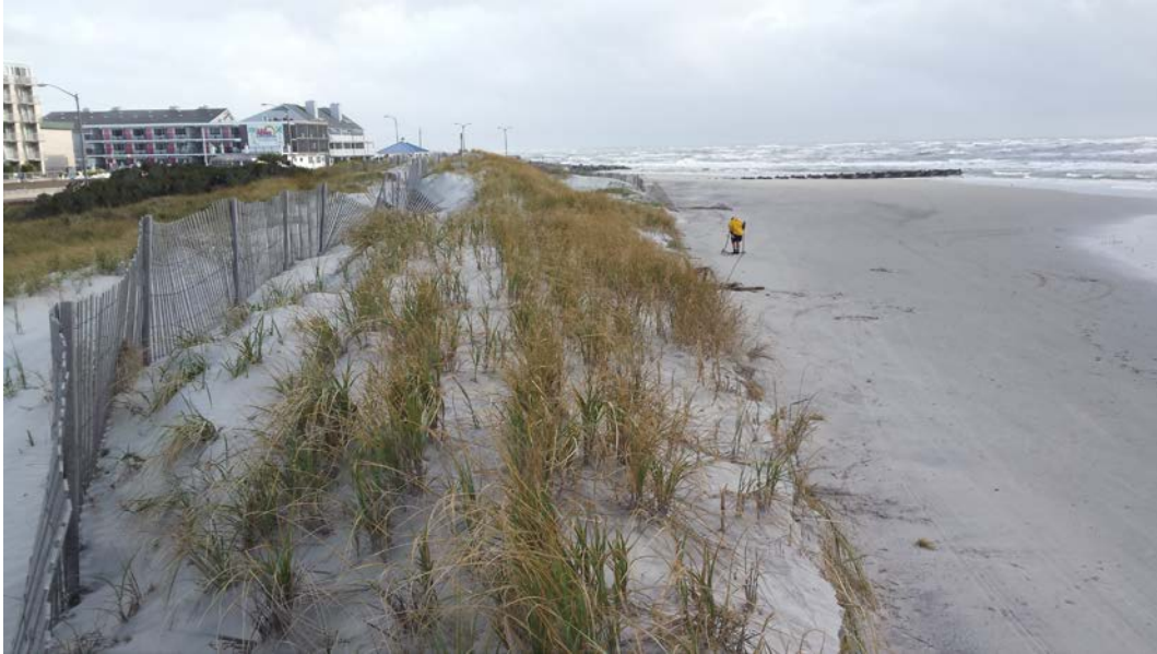
Figure 7. View from 5 th Avenue looking north taken on October 3, 2015 following the northeast storm events and Hurricane Joaquin. A significant scarp in the seaward duneface is shown along with recreational beach elevation and shoreline losses observed.
