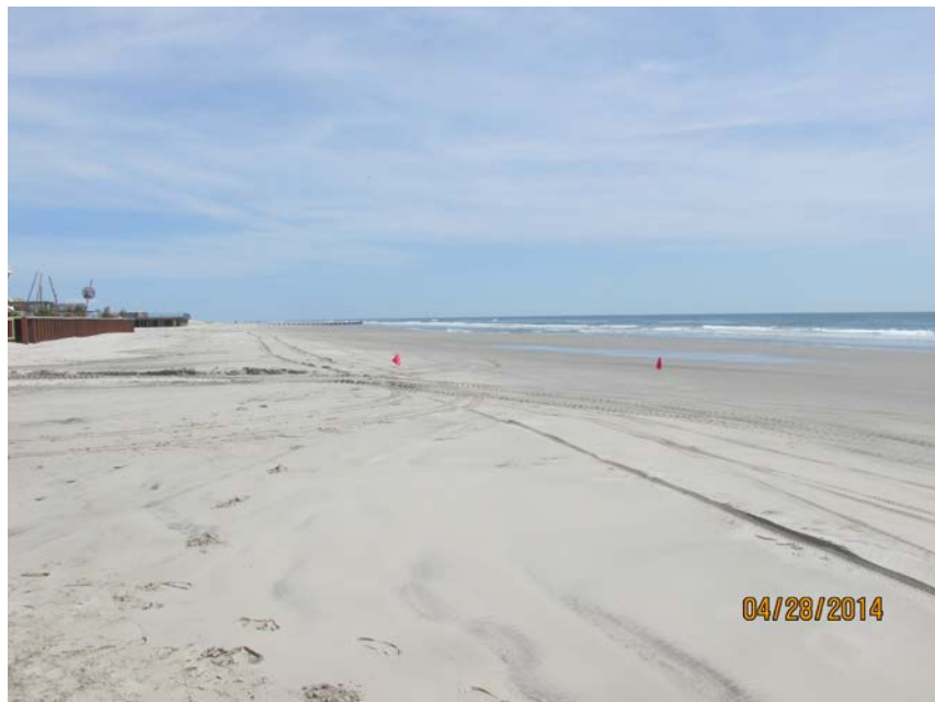
Figure 22. View to the north taken on April 28, 2014 from near 26 th Avenue showing the extent of dune erosion and repositioning of the initial dune system landward of the eastern-most portion of the southern piers. As a direct result of the initial position of this protection feature being constructed seaward of the piers, by February 2014 the majority of the dune system had eroded.
