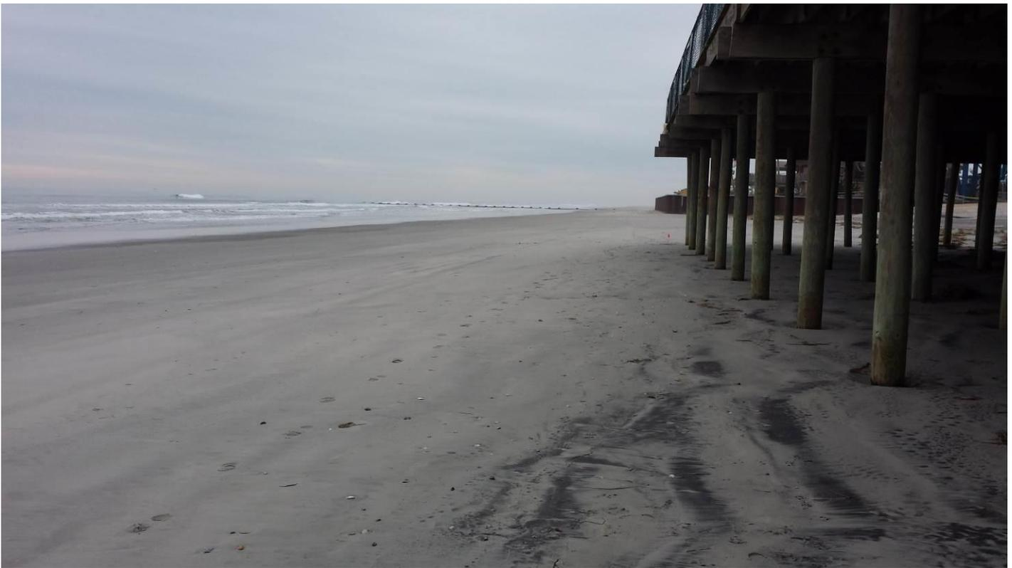
**Figure 20.** A close up view of the beach at the very seaward end of the timber pier indicating that no dry beach or dune feature remains at the pier's end (March 2017). Visible between the pier pilings is the re-positioned dune between this pier and Morey's Surfside Pier.
