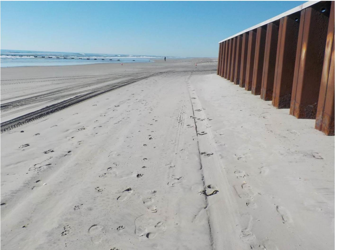
**Figure 25. View to the south taken on October 20, 2017 near 26<sup>th</sup> Avenue following the summer season demonstrates that sand does not accumulate above normal high tide because wave reflection off the wall moves it back into the swash and eventually south into Wildwood. There is a significant bar offshore, but that material has yet to migrate onto the beach.**
