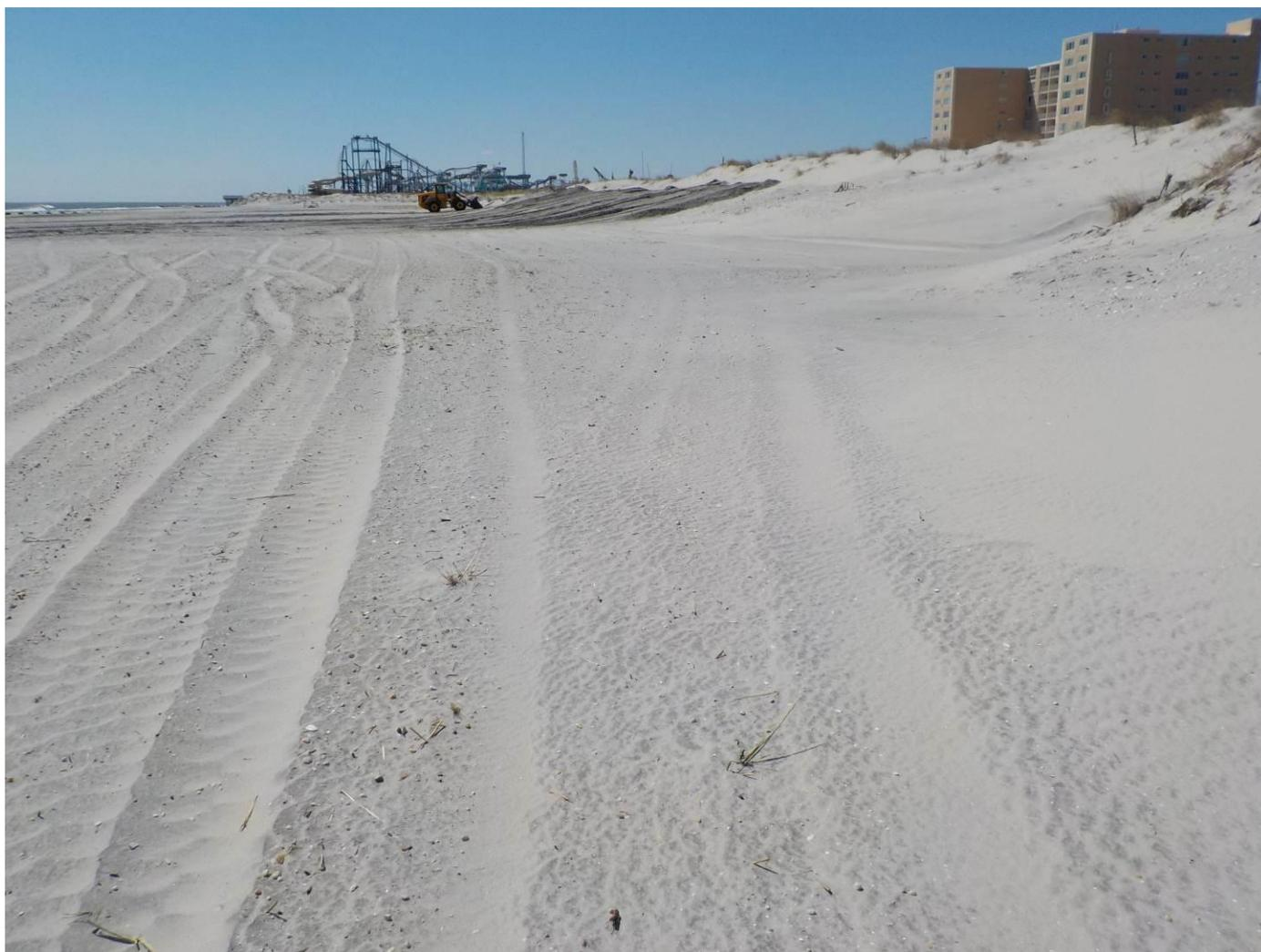
**Figure 14. View to the south along the seaward dune toe March 23, 2017 as work was in progress pushing sand onto the seaward dune slope. Sand accumulated here during the year adding to the stability.**
