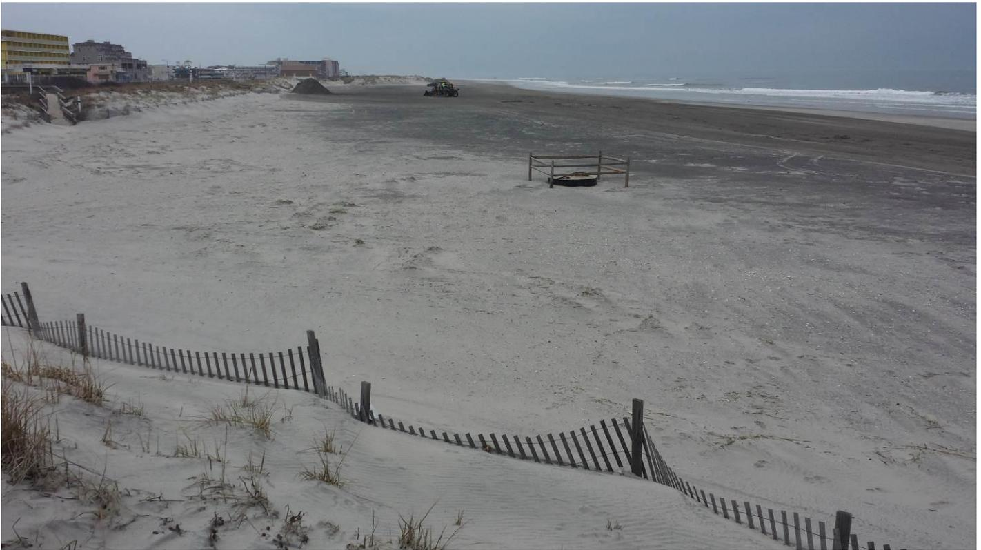
**Figure 17. View to the north taken from the dune crest at 21<sup>st</sup> Avenue on March 23, 2017. Sand continued to accumulate at the dune fencing installed after Hurricane Sandy and work in the distance was underway to recover sand from the beach berm to use on pedestrian beach access paths and at the dune toe where needed.**
