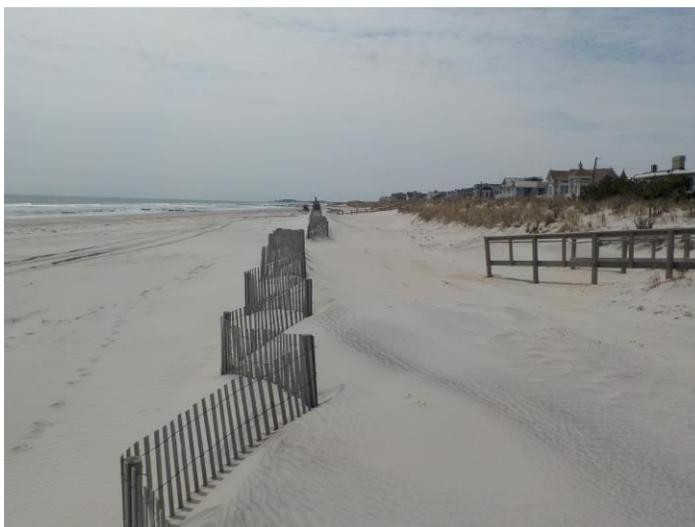
**Photoplate 4b - Photo taken April 9, 2018 shows the winter’s accumulation of sand around the new fence. This beach changed very little during the year.**
