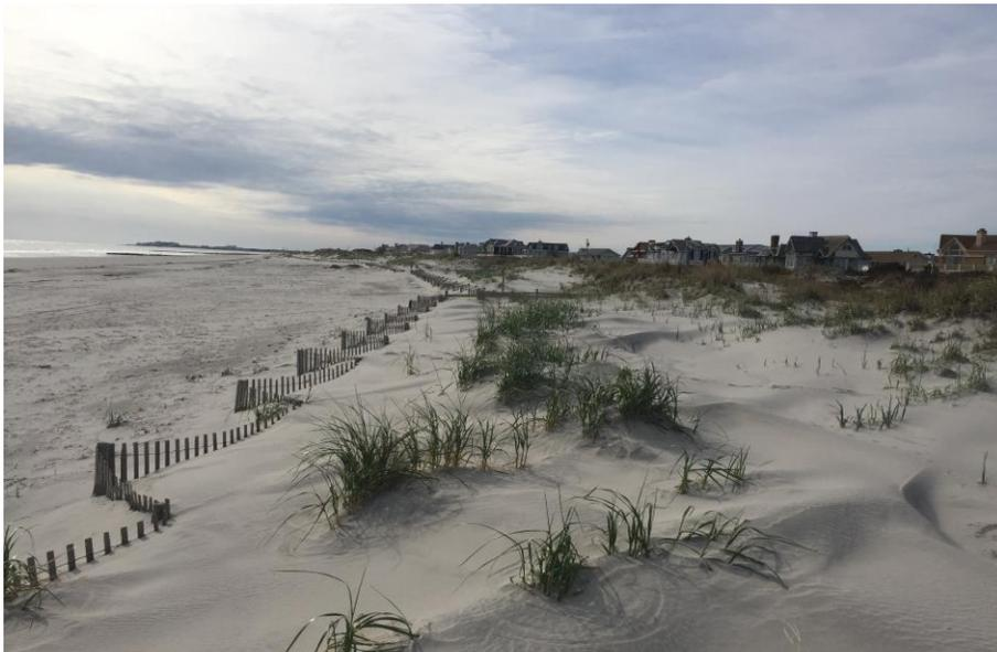
**Photoplate 7c – Photo taken November 8, 2018 showing the well-established dune and the added material deposited landward of the fence row.**
