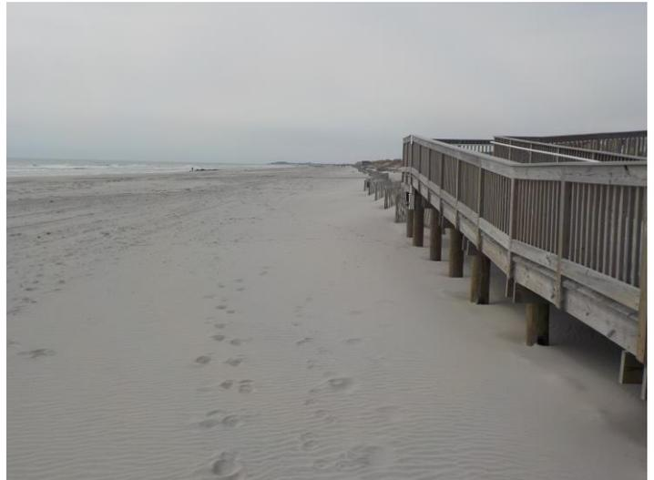
**Photo 3b – The April 9, 2018 photo shows the entrance ramp positioned at the dune toe alignment with a dry beach seaward.**
