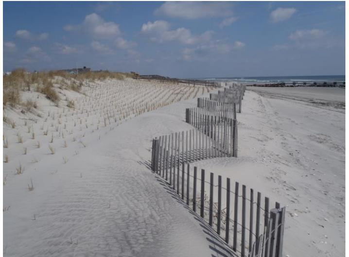
**Photoplate 6b - Photo taken April 10, 2018 shows the newly planted grass with wind-deposited sand accumulating around the fence.**
