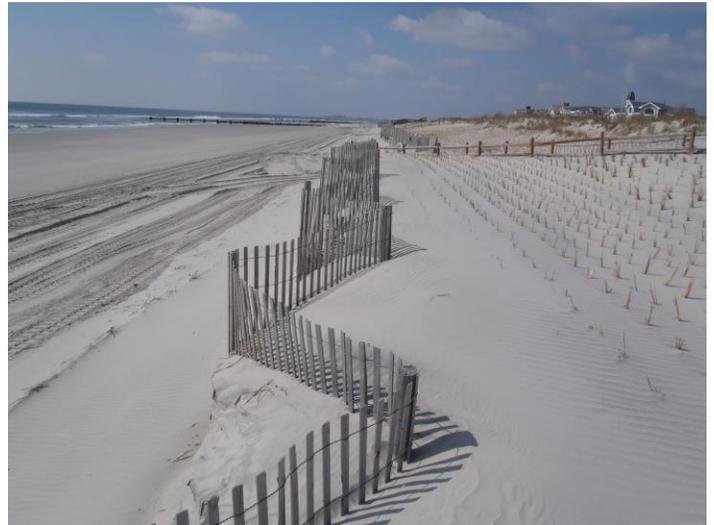
**Photoplate 5a – The October 3, 2017 photo shows the sand fencing installed to help protect the dune toe. The beach width was less than following the fill.**
