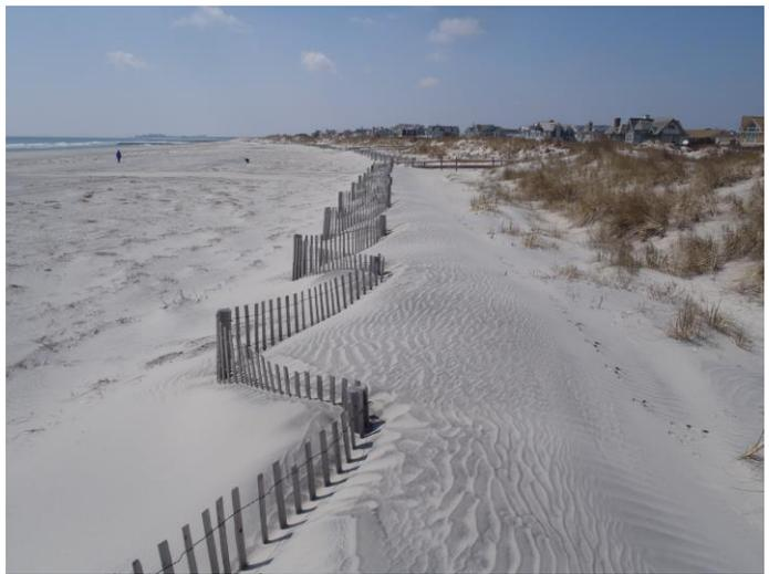
**Photoplate 7a - Photo taken October 3, 2017 shows sand accumulation around the fencing as wind deposition added to the dune.**
