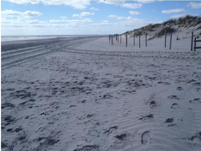
**Photo 1a – Photo taken October 3, 2017, this was the fall after the beach restoration where dune fence posts had been installed for a new dune toe fence.**
