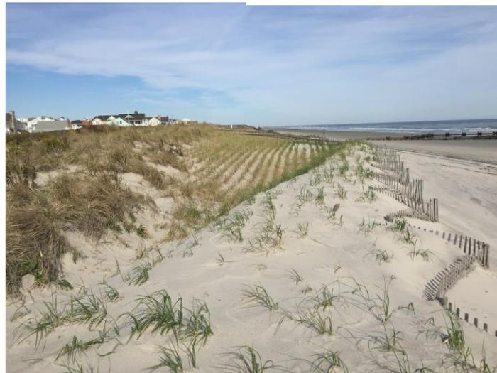
**Photoplate 6c – Photo taken November 8, 2018 overlooking the accreting foredune encroaching onto the planted project dune slope with its neat rows of grass established. The fencing is nearly buried with new sand from the beach.**
