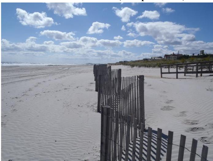
**Photoplate 4a - Photo taken October 3, 2017 showing sand fencing placed seaward of the dune toe.**
