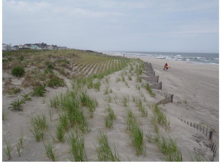
**Photoplate 6a – The November 8, 2018 photo shows the accreting foredune with new natural plants springing up seaward of the rows of plants added in 2017.**
