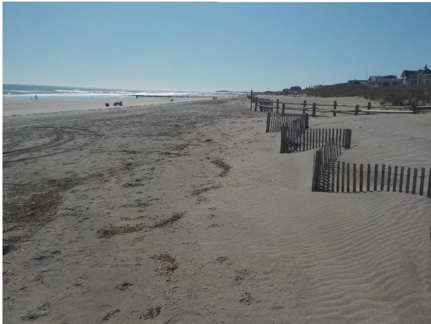
**Photoplate 4c – Photo taken October 14, 2019 showing sand continuing to fill the 4-foot high snow fencing creating a new foredune. The beach width was sufficient to provide the supply.**
