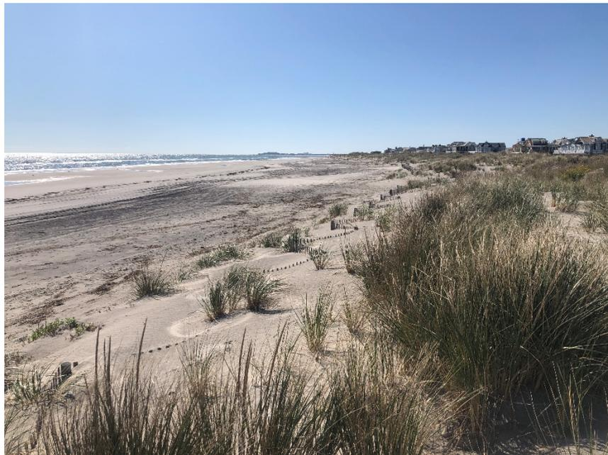
**Photoplate 7c – Photo taken October 15, 2019 finds the fencing placed in 2017 completely buried and luxuriant dune grass growing across the feature created since the fence was built.**
