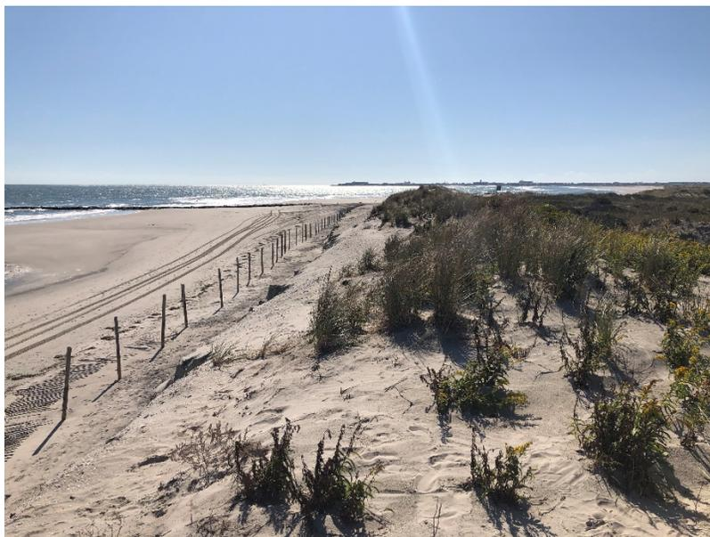
**Photoplate 8c – The photo taken October 15, 2019 following another episode of dune toe erosion generating a 4-foot scarp in the toe. The sand supply is not sufficient to maintain even a minor storm proof dune.**
