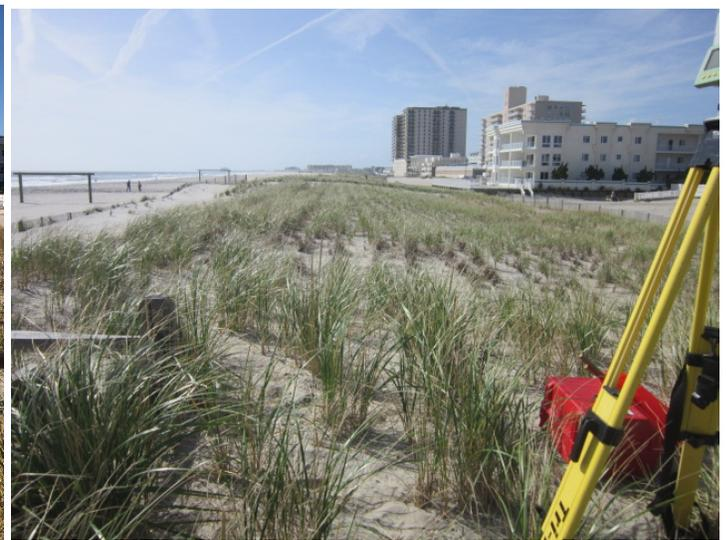
The Benson Avenue site is located approximately one mile south of the end of the original USACE project in Ventnor. The left photo taken November 13, 2019 shows the post project dune and beach configuration with a wide dry beach berm and newly planted dune and installed dune fence. By October 19, 2020, the dune fence is accumulating sand and the vegetation flourishing on the crest. Following construction, the beach has remained relatively stable throughout the study interval.
