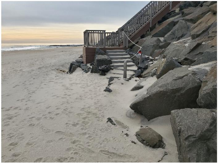
This site is located on the boundary between the bathing complex and private homes which extend south of the location. The Jan. 7, 2020 view was shot at the toe of the rock revetment built post-Sandy at the site with some wind deposition generating an incipient dune (left view). The 4-foot high fence has been buried. The right hand side photo shows additional sand deposition at the rocks with fewer steps exposed.
