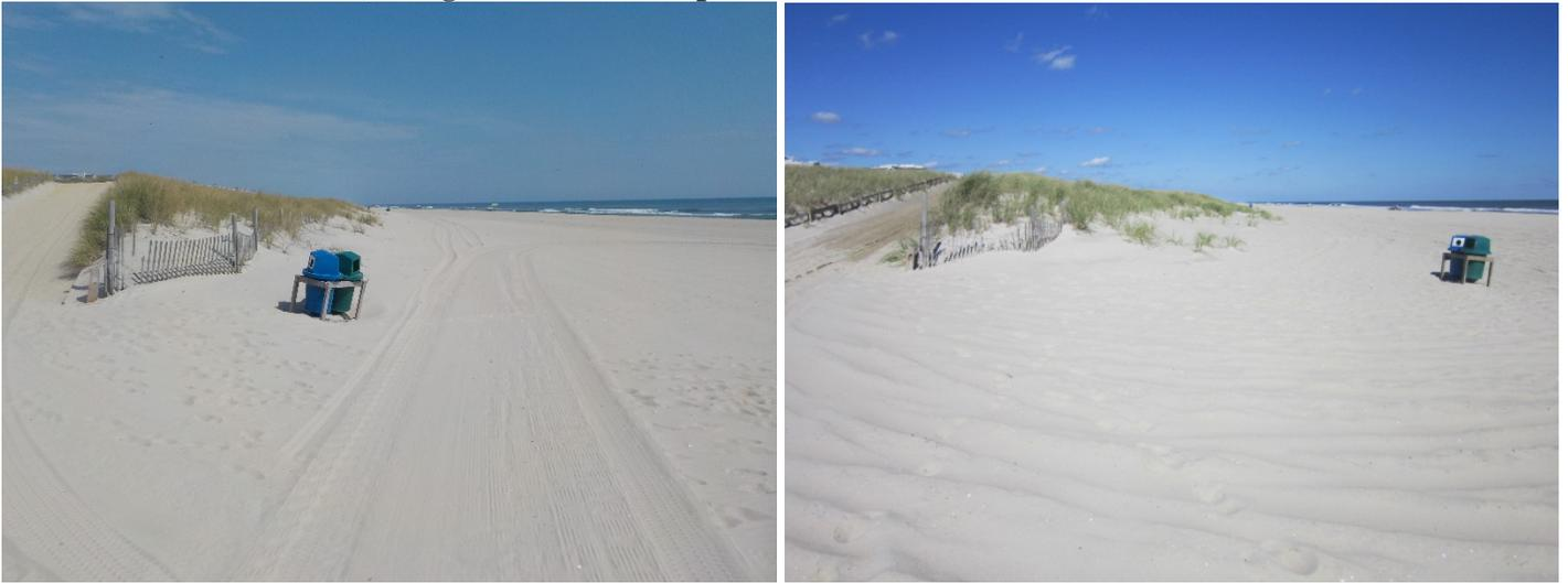
At the Township’s 81<sup>st</sup> Street profile there was a modest accumulation of sand at the seaward dune toe between 2019 and 2020 (left photo taken September 12, 2019 and right taken September 30, 2020). The engineered dune has remained at the same elevation since it was constructed in 2015.
