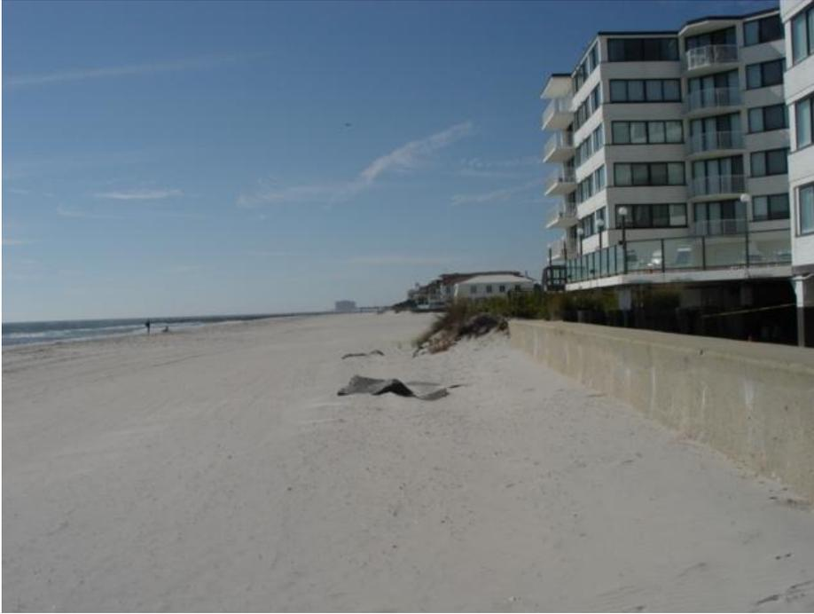
The Longport site is about 15 blocks from the terminal jetty to Great Egg Inlet at 11<sup>th</sup> Street. This October 22<sup>nd</sup> 2007 photograph shows the concrete seawall with sand ramped up to within three feet of the crest. Note that the armor stone seaward of the wall's base just barely appear. Insufficient beach width exists to establish a dune along this segment of shoreline.
