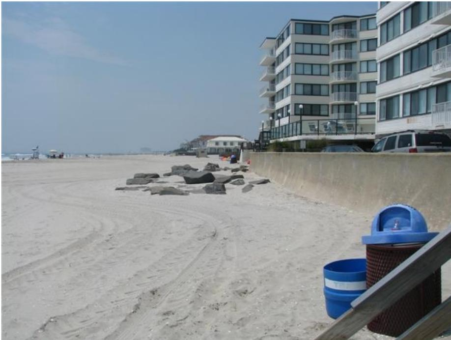
By the spring of 2008 (June 27<sup>th</sup> 2008) the wall height had increased to 5 feet as sand was removed, exposing the tops of the surface rocks to the south of the access stairway. Since the Federal project's completion, this beach has gained 29.41 yds<sup>3</sup>/ft. and the shoreline advanced seaward by 12 feet. The sand volume gain is considerably larger than seen in the past.
