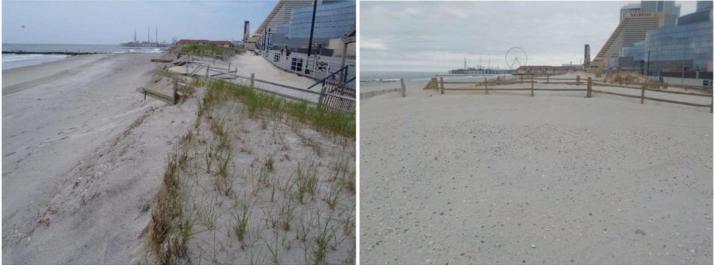
This profile site is located near the Absecon Inlet south jetty. The June 21, 2016 (left, view to the south) shows a scarp cut into the dune with damaged fence and steps remaining at the beach access path. The right photo (taken December 22, 2017) shows the restored beach and dune following the USACE 2017 maintenance project.
