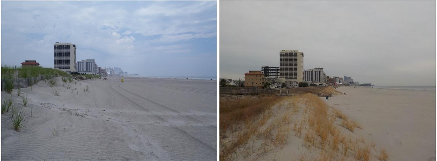
This site lies near the middle of the initial USACE shore protection project on Absecon Island where erosional loss is minimal. On the left (June 21, 2016) looking north along the seaward dune toe sand is collecting along fencing placed relatively recently. The photo on the right taken December 20, 2017 shows that sand accumulated at the fence now completely buried, dune grass colonized the seaward slope to the toe.
