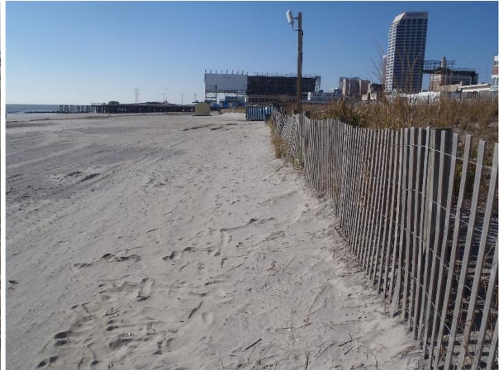
This location is also within the Absecon Island Federal shore protection project just south of Steel Pier. The left photo, taken December 22, 2017, shows the beach under construction. Photo shows the beach and seaward dune toe one-year post construction (November 21, 2018). At this location, the project beach is relatively stable and supports the established dune.
