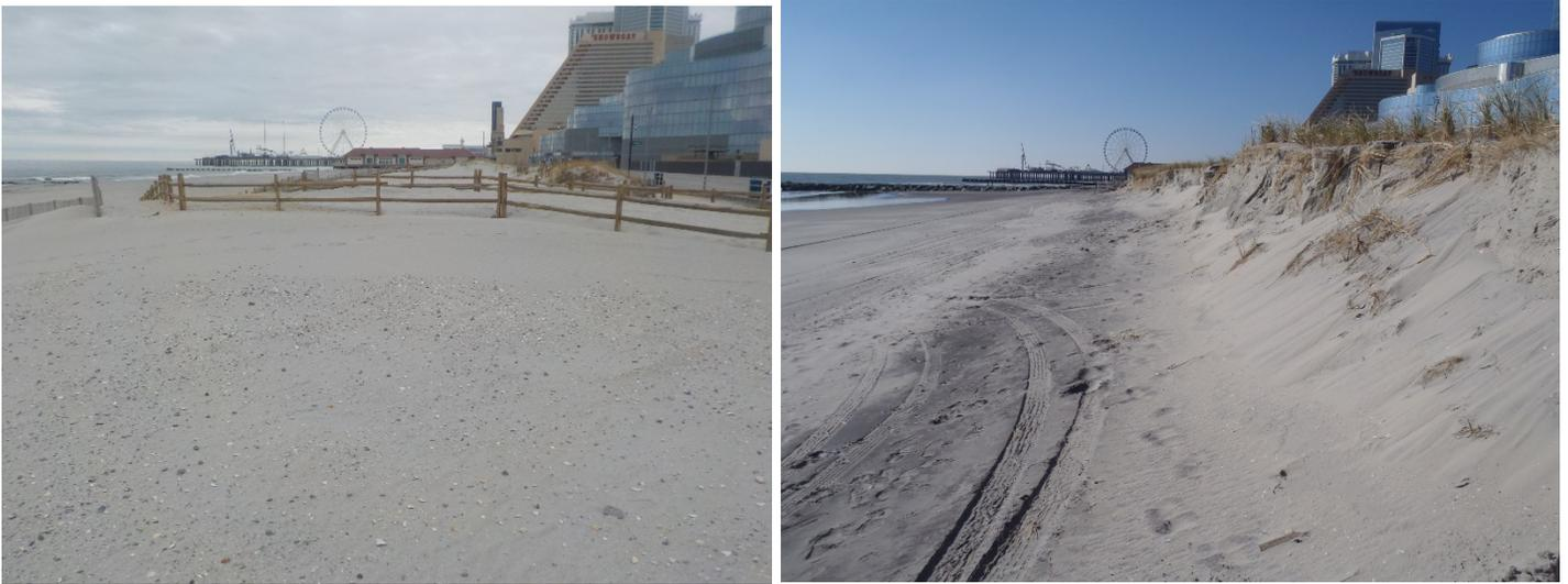
This profile site is located near the Absecon Inlet south jetty. The left photo (taken December 22, 2017) shows the restored beach and dune following the USACE 2017 maintenance project. By November 21, 2018 (right photo) erosion had lowered the beach berm elevation reduced the overall width that allowed storm waves to cut into the seaward dune slope. This site remains an erosional hotspot for Atlantic City despite rehabilitation and modifications to the adjacent rock groins.
