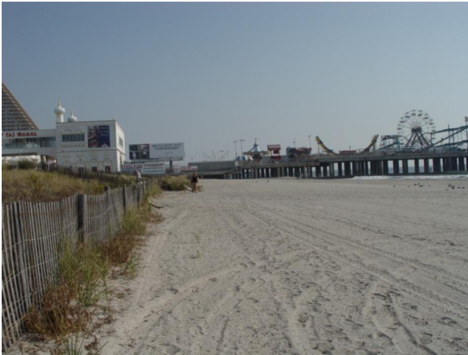
Figure 210. The North Carolina Avenue beach remained stable through the summer of 2007 with material slowly added to the dune as the vegetation matured. The beach width south of the pier did not change much and storm damage was absent as of October 17, 2007.
