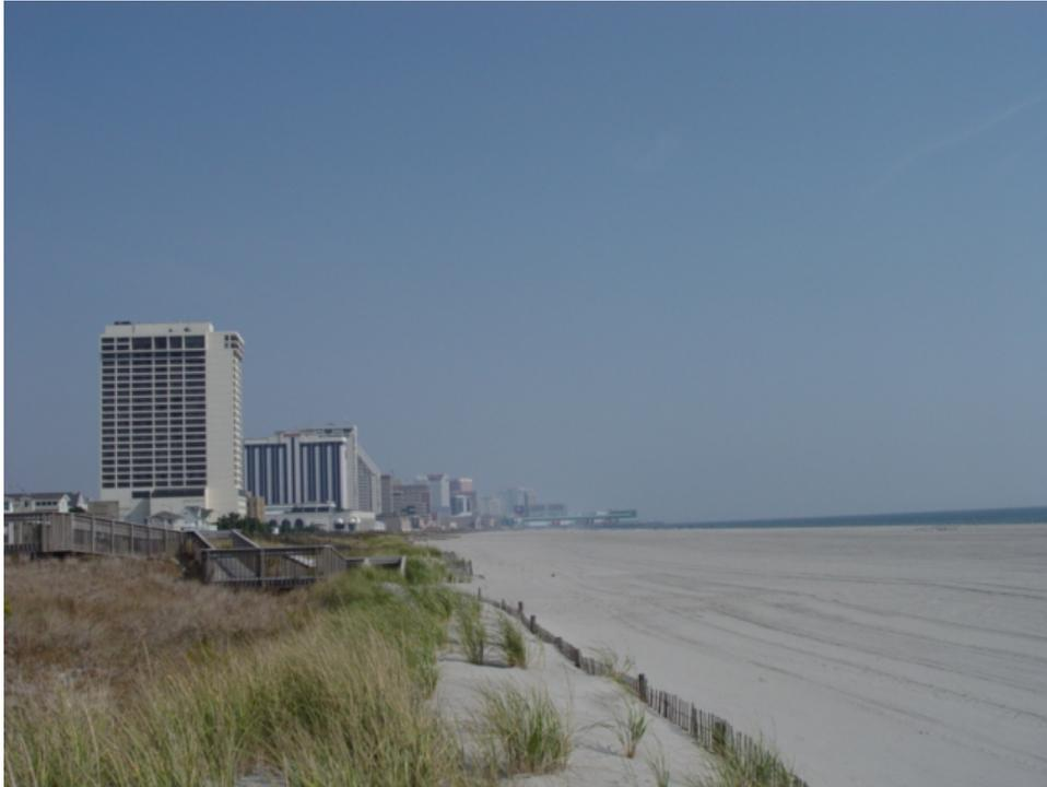
Figure 215. By October 2007, the dunes had accumulated additional sand at the line of the original fencing. This shows to the left as very vigorous grass and a nearly buried line of sand fence. The beach width and height has remained relatively stable, as designed and built during the project's construction.
