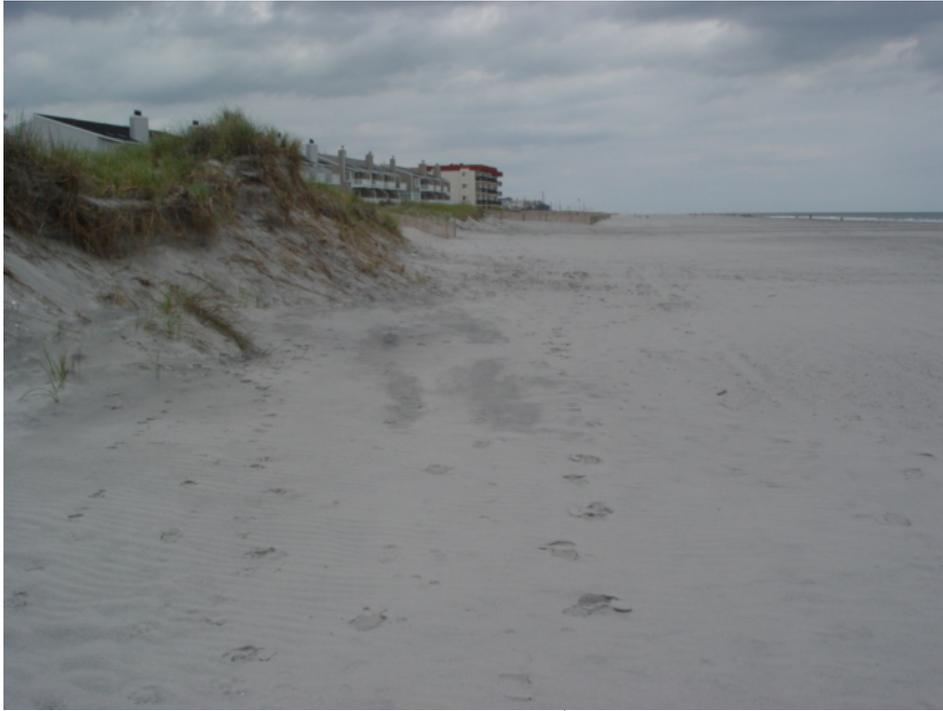
Figure 195. This site is at the northern end of development in Brigantine, but at the southern end of the original 1997 beach nourishment project. The beach has retreated from the “as-built” width, but remains in far better condition than it was prior to the 1997 project. Work by the City and State in 2001 restored this beach then Federal project undertook the initial ACOE-sponsored work. This finished in 2006 extending reconstruction 10 blocks further south with modest sand volumes.
