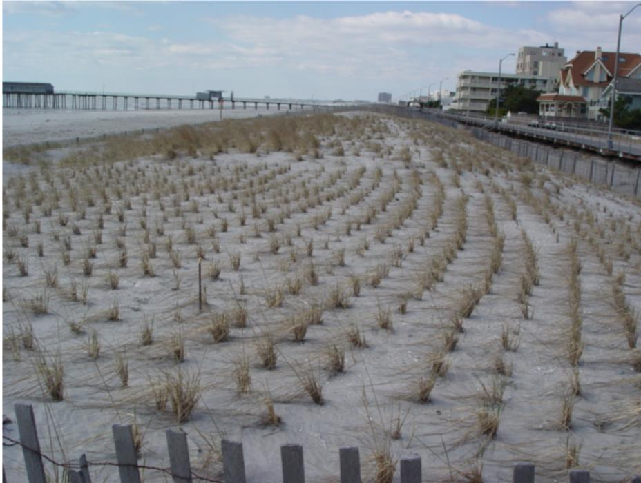
Figure 218. The Dorset Avenue site in Ventnor City received a new dune, plants and a much wider beach in 2004 as part of the federal project. The photo shows the recent plant placement pattern and the wider beach as built, which continues south towards the Margate City border.
