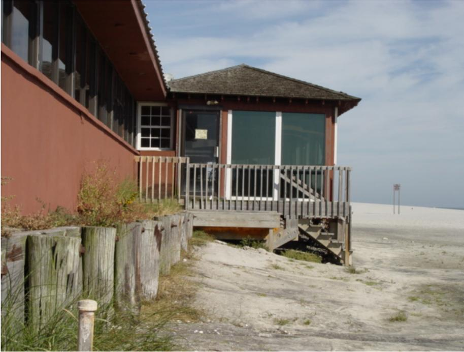
Figure 202. This picture shows the relationship between the timeshare development and the beach. The aging bulkhead is the only shore protection feature present, in previous storm events the building to the left filled with sand. The structure in the center was not present during the December 1992 northeaster. The absence of a dune and flat low profile of the beach could allow wave impacts against the bulkhead from a significant storm event that would have serious consequences for this building.
