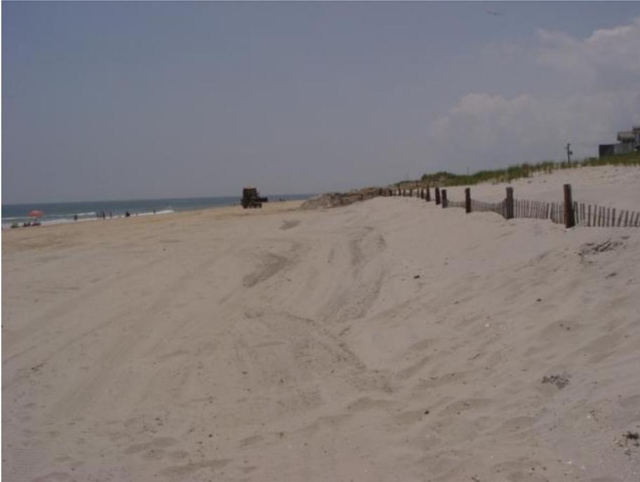
The June 11, 2007 survey followed the completion of truck hauling about 80,000 cubic yards of quarry sand to the beach between 10<sup>th</sup> and 17<sup>th</sup> Streets. The slight yellow cast to the dry beach is the clue that this occurred.
