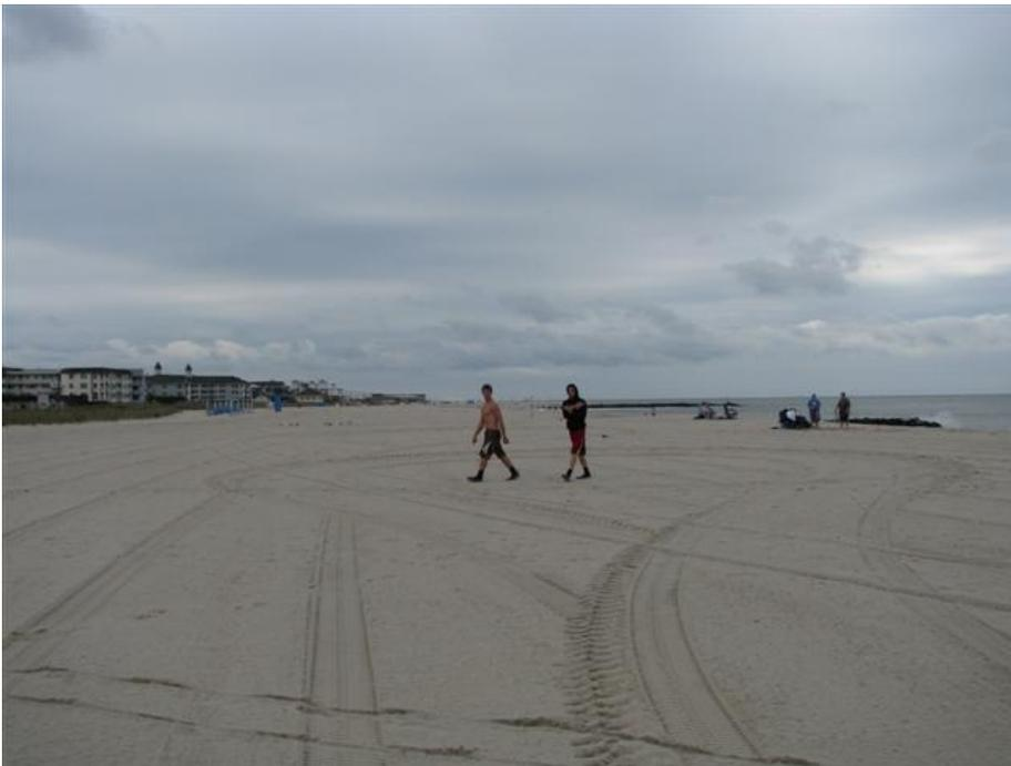
By September 10, 2008 the beach was in similar condition since there has been very few storms. The groin in the picture is a little more exposed, but not significantly so. The survey data indicates a minuscule sand volume change of  $0.04 \text{ yds}^3/\text{ft}$ . coupled with a 17-foot shoreline advance.
