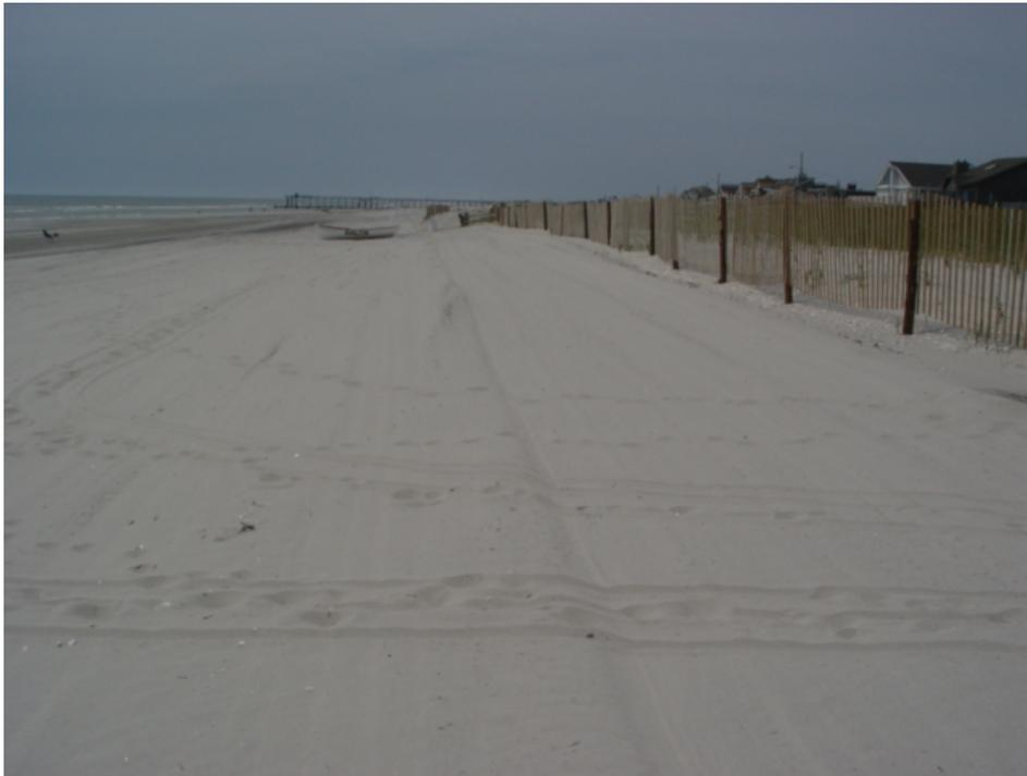
Figure 267. Looking south from the 23<sup>rd</sup> Street site the beach and fence are new from the recently completed back passing of 55,000 cubic yards of sand from the mid-island beach. Trucks hauled the sand back and placed in it a huge ridge that was graded into the profile shown as survey 32. The picture was taken May 25, 2006.
