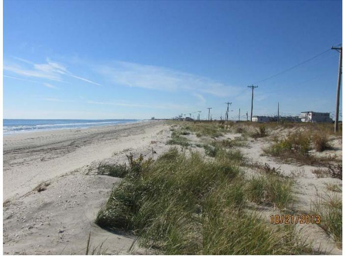
The dune here at the 1<sup>st</sup> Street location consists of a geotextile core covered by sand. The pre- H. Sandy photo (left, taken October 17, 2012) shows a berm higher in elevation than the photo on the right (taken October 21, 2013). The dune remained intact and most of the sand was transported either southward or into the nearshore.
