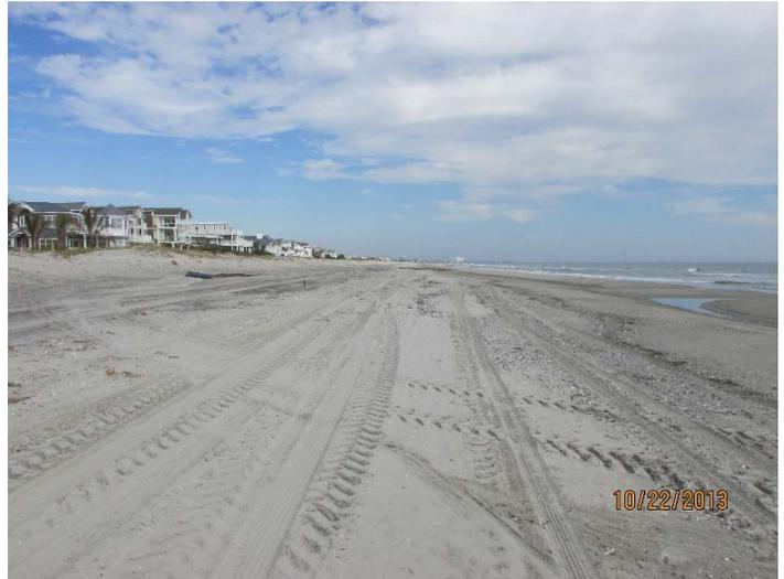
The 80<sup>th</sup> Street location was included in state/local beach fill and contained a newly created dune via sand fencing (left photo taken October 22, 2012). Following H. Sandy, sand that washed inland was hauled back to the beach and placed at the toe of the eroded dune. The photo on the right (October 22, 2013) shows a low-elevation berm and an exposed low-tide ridge/runnel as the nearshore bar has moved landward.
