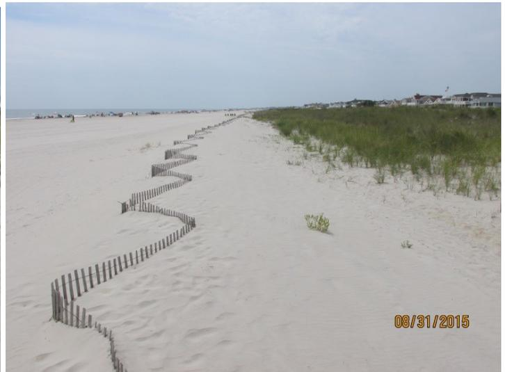
The comparison photos to the south (left taken September 5, 2014 and right photo taken August 31, 2015) show minimal changes to the dune vegetation with respect to the location of the dune fencing. This profile is located nearly in the center of the island and continued modest volumetric gains for both 2014 and 2015.
