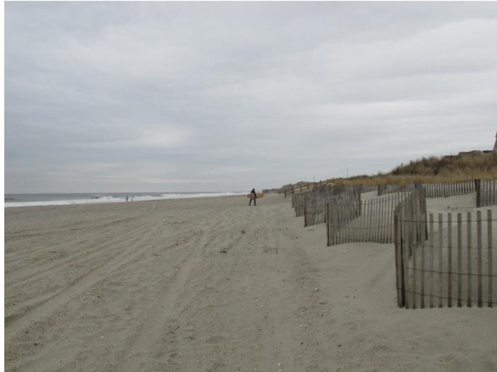
The 9<sup>th</sup> Street site is located near the Townsend's Inlet south jetty. There was no wave attack on the properties due to Sandy and the beach was restored during 2013. The dune fence shows a considerable accumulation at the fence with a narrow beach beginning to emerge to the south by September 15, 2014. The right photo taken, on October 7, 2015, followed an Avalon-funded beach restoration in 2015 augmenting the post-Sandy federal work in 2013.
