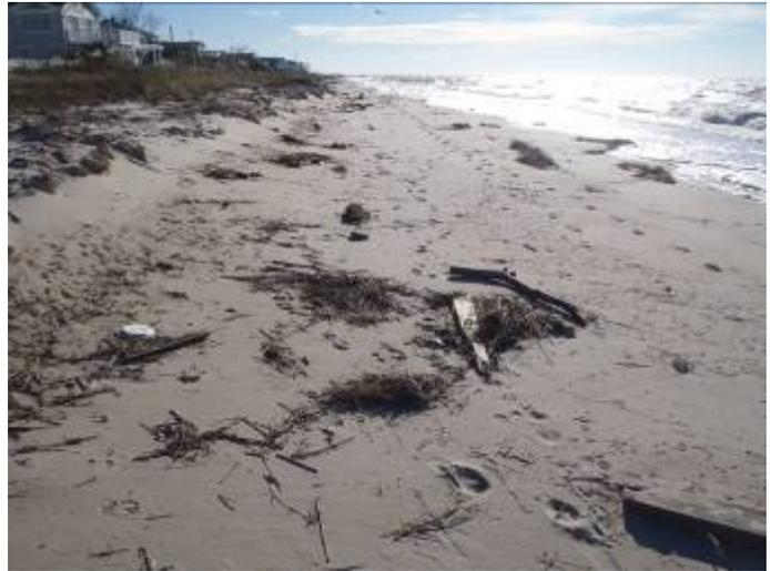
The left view was taken March 7, 2012 looking south along the beachfront. By November 9<sup>th</sup> the storm impact was found to have eroded the beach into the toe of the dune reducing the beach elevation and creating a minor scarp. The height of the uplands bluff prevented local wave or tidal flooding.
