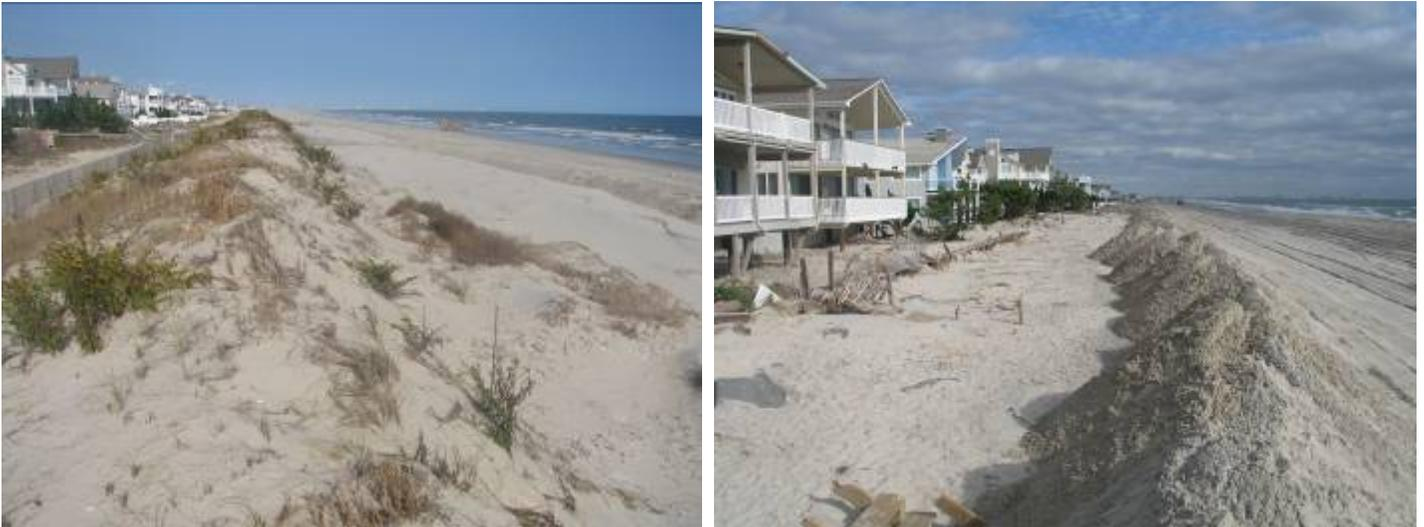
The left photograph was taken October 26, as Sandy was approaching NJ. Machines were deployed pushing up a ridge of sand seaward of the existing dunes at this site. Sandy overwhelmed the shore protection, jumped the old bulkhead and washed well inland producing damage and flooding. The right picture was taken November 6<sup>th</sup> and shows recent bulldozing efforts to provide a small measure of protection for homes with nothing between them and the sea.
