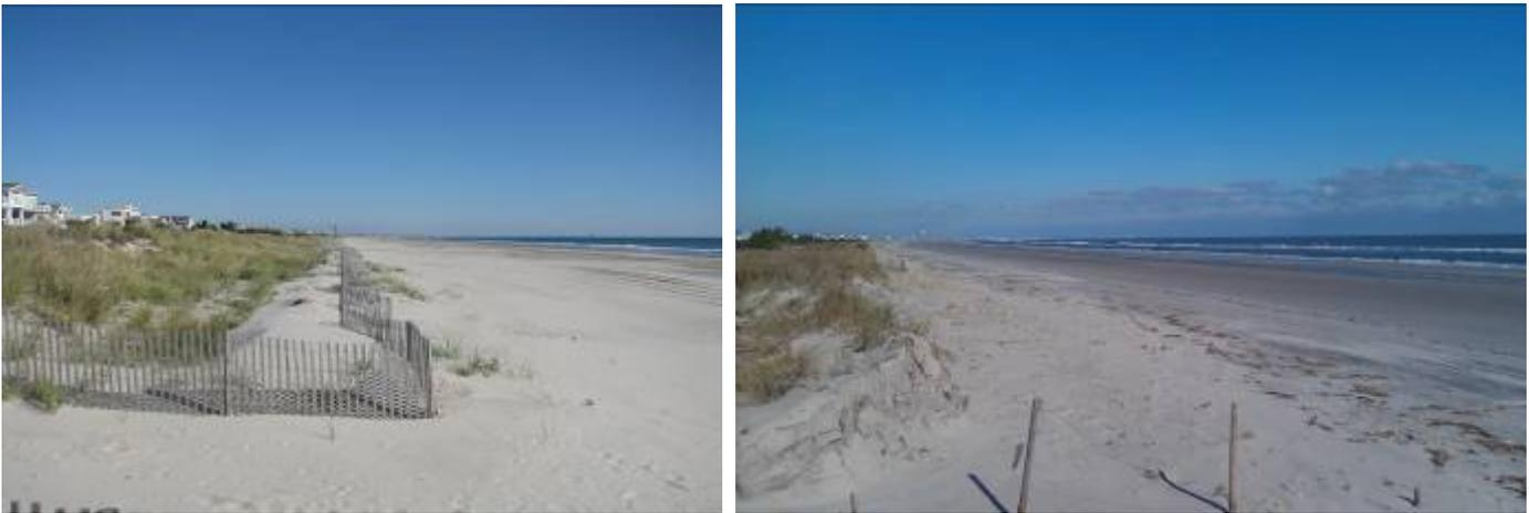
On October 22, 2012, the beach was relatively wide and dry with a decent new deposit of sand along the recent fencing installed at the seaward toe of the dune system. After Sandy on November 14, 2012 the beach was lower in elevation, all the fencing was missing and sand was pushed back into the dunes, up the seaward slope.
