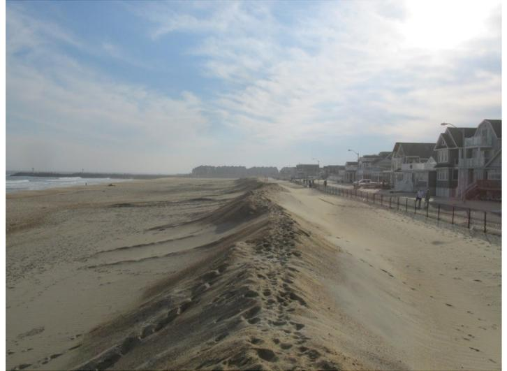
By May of 2014 the beach had 82.26 yds<sup>3</sup>/ft. in new sand added by the USACE resulting in a 113-foot shoreline advance. The Dec. 22, 2014 view on the left shows a single fence and no dune, while the Dec. 11, 2015 view on the right shows that the municipality had pushed up a sand ridge as a winter “dune”. This precludes any sand building around the fence line.
