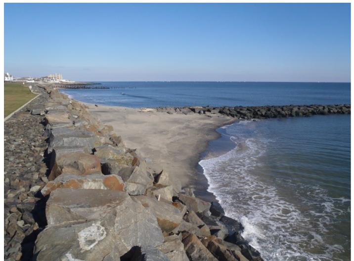
This profile is located between two rock groins that limit sediment movement. This area has never received sand from direct beach nourishment. The photo on the left (taken November 21, 2014) shows the deposit of sand derived from the storm erosion of the bluff. By December 4, 2014 sand moved offshore and adjusted lower at the rocks.
