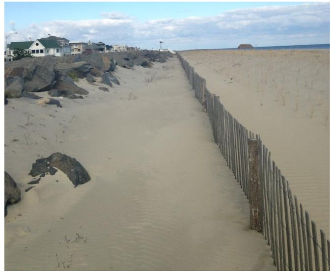
This site has the worst erosion history of any site in Monmouth County. The left photograph Nov. 25, 2014 shows the completed work by the USACE after one year following a 180-foot berm crest retreat. On the right the existing beach has narrowed further with a single straight line of snow fencing in place to start a dune on site as of Dec. 24, 2015.
