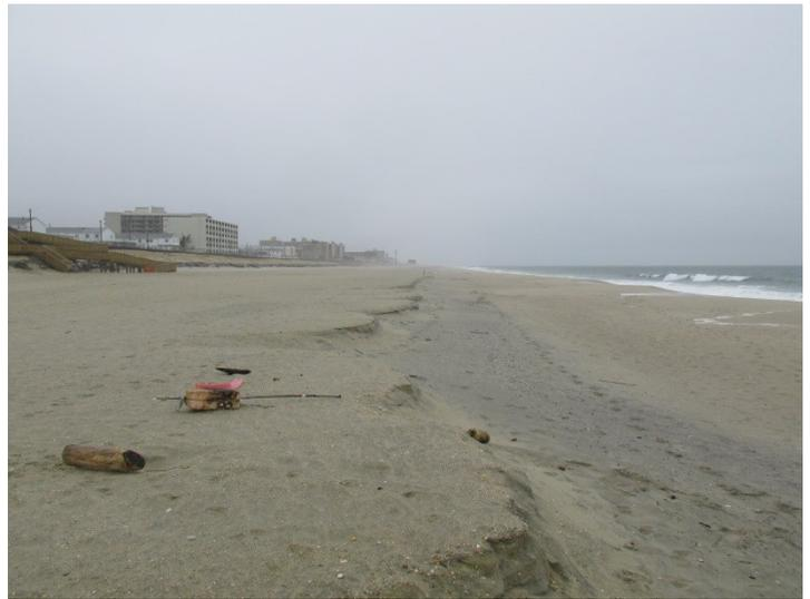
This site is located near the southern limit of the Federal beach nourishment project. The fencing keeping people out has been removed with the walkway moved onto the southbound road once part of Ocean Avenue. The December 3, 2014 view shows artwork on one revetment rock re-deposited on the seawall, looking over the new federal beach. The December 16, 2015 view on the right illustrates berm erosion followed by bar welding onto the beach generating a new berm position.
