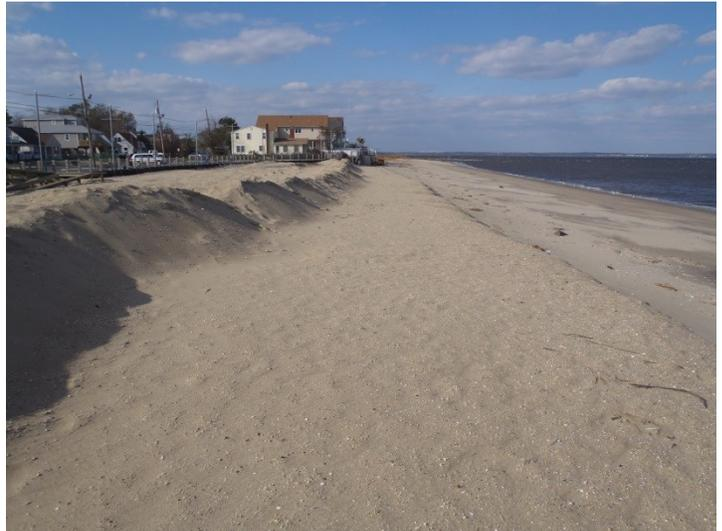
This site was enhanced by adding slope protection to the eroding uplands bluff prior to Sandy. The photograph on the left shows the shoreline on October 7, 2014 following the ACOE project’s completion. The right picture was taken November 13, 2015 where scarping has cut into the “as-built” profile and sand was pushed up to provide storm protection.
