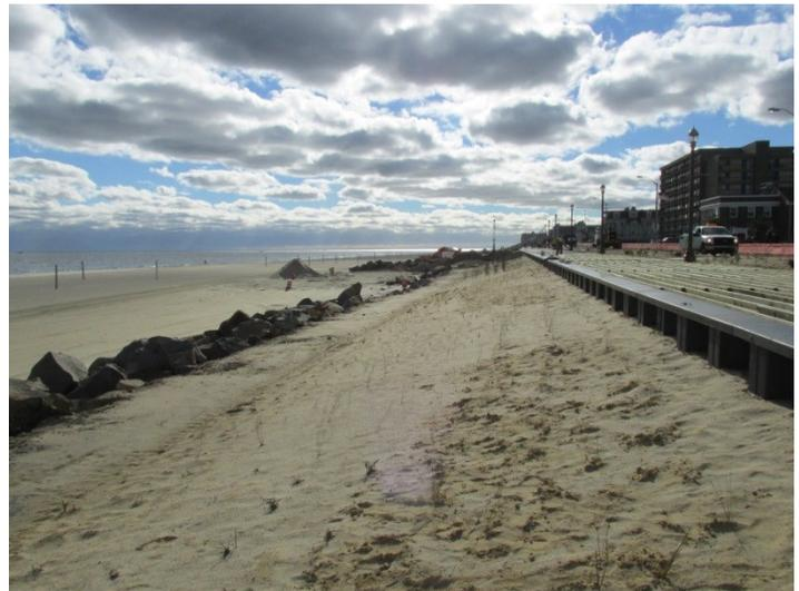
It appears as if the City has moved the pedestrian walking zone onto half the remaining southbound roadway that once existed here as a dual road as Ocean Avenue plus the boardwalk in 1960. The ACOE activity is very evident in the left picture taken December 3, 2014 (complete as of survey #48). By December 16, 2015 a new roadside bulkhead was installed and a graded slope to the rock revetment completed the storm damage repairs. The beach remains in good condition.
