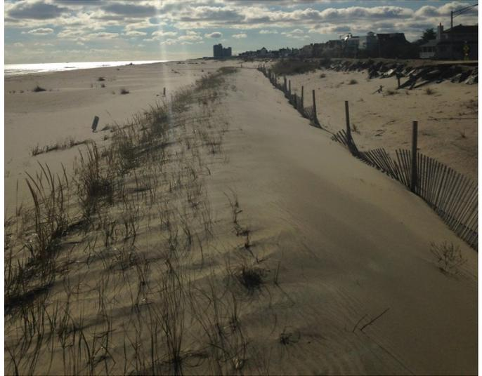
The restoration by the USACE had been completed in the left photo taken November 25, 2014 for a year, with the addition of 101.64 yds<sup>3</sup>/ft. to the profile's cross section. A small dune was added by the summer of 2014 as sand was redistributed somewhat at the water's edge and enhanced by December 24, 2015 with wind transported sand.
