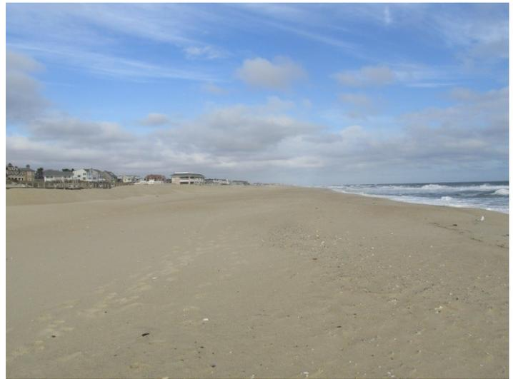
By December 11, 2014 (left) the USACE had added 40.47 yds<sup>3</sup>/ft. in new sand advancing the shoreline by 13 feet. The right view on November 29, 2015 shows the wide beach with an active surf zone breaking on an offshore bar.
