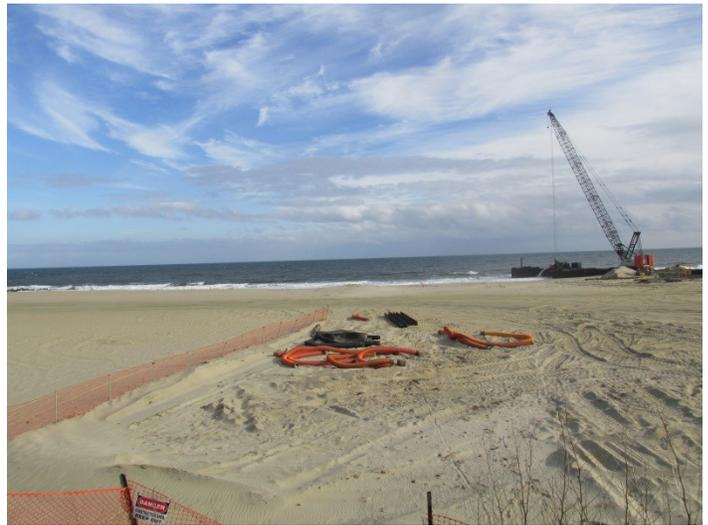
The Darlington site has a small sub-aerial beach contained between two larger groins. The upland bluff was eroded significantly during Sandy and added to the beach sand. By November 14, 2014 (left) natural recovery added 26.32 yds<sup>3</sup>/ft. back to the beach with some reconstruction of bluff protection structures. A year later (Nov. 30, 2015) the USACE project was underway adding dramatically to the beach with additional groin work in progress as well.
