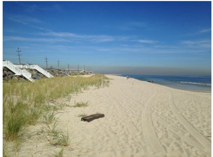
This site is near the northern limit of the initial Federal shore protection. The left side shows the results a year after the placement of 40.12 yds<sup>3</sup>/ft. of new sand and a new dune on the beach by Oct. 8, 2014, while the right side (Sept. 16, 2015) shows how well the dune grass developed and added material to the dune.
