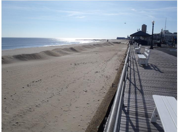
This site in Allenhurst was the starting point for Phase III USACE work in 2015. The left side view (May 18, 2016) to the south includes Loch Arbor and in the distance, Asbury Park. The right side view from the top of the old concrete seawall shows the storm ridge pushed up to mitigate wave damage as of December 7, 2017.
