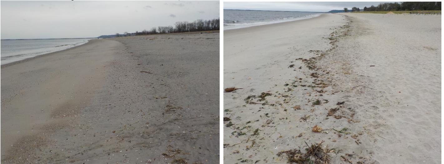
This site was enhanced during 2014 by the NY USACE. The April 1, 2016 view on the left along the beach to the east shows the established profile. The right picture was taken September 18, 2017 confirming the minimal changes documented by the surveys. Sandy Hook lies at the horizon in the distance.
