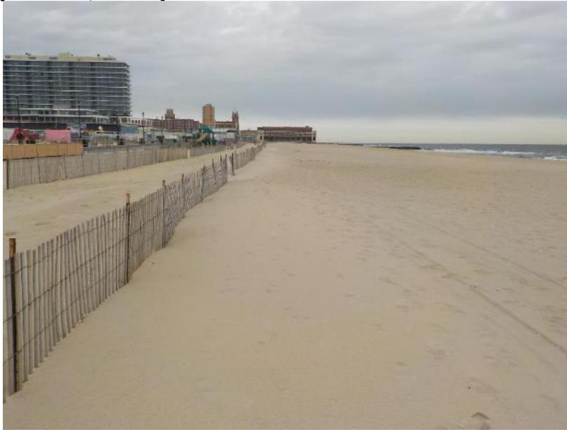
The beach remains at a decent width with minor berm retreat. There is no bar offshore as of the end of the initial year of surveying. A small, unvegetated “dune” is now present between two rows of fencing.
