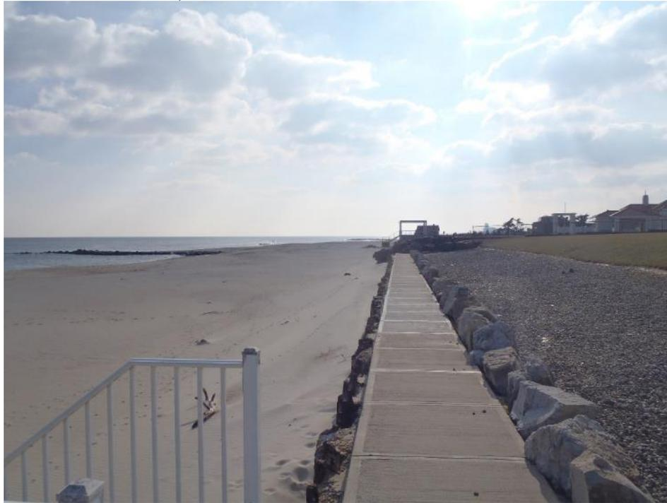
The survey shows a 200-foot wide beach with a small terrace offshore, no dune and some readjustment in the cross section since the fill was complete. Most change occurred in the berm and with bar migration offshore.
