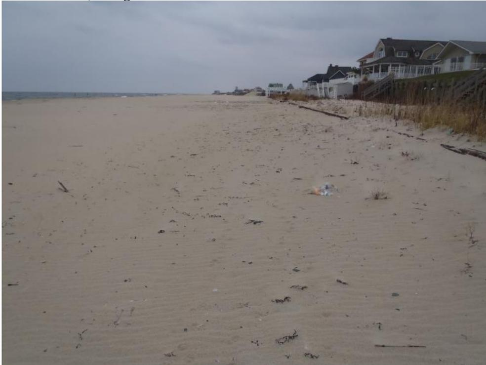
This site retains a wide beach with a significantly built up berm leaving 260 feet of elevation 10.0-foot beach remaining. The bar system offshore has been present since the initial survey. There are no dunes along this Elberon bluff segment.
