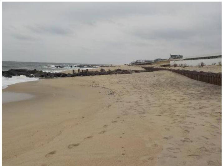
This site is located on the highest point along the bluff shoreline. The photo on the left (taken December 12, 2017) shows the new beach after some adjustment. The vertical bulkhead just shows to the right side. By December 2018 the four pilings and a rock that show on the left are part of a fully exposed groin with the bulkhead more extensively exposed as well.
