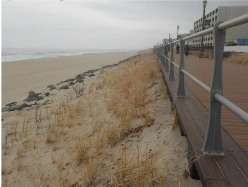
The rock revetment is followed by a 170-foot wide beach to the berm and a beachface slope to a terrace about 4 feet below the datum with a small bar present. Over the past year, this bar has grown larger.
