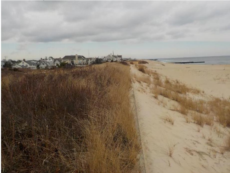
The extraordinary dune elevation is because the National Guard shooting range ends at its landward side, so the extra height was added to stop bullets. This beach is off limits to the public, about 150 feet wide with an offshore bar.
