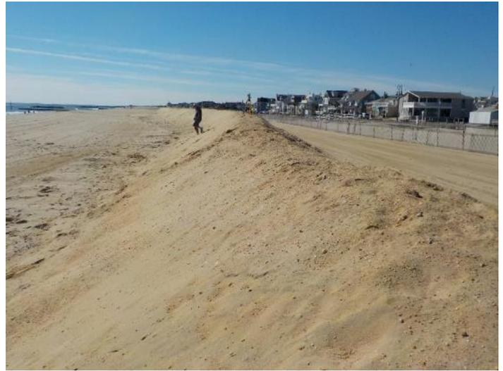
The November 7, 2017 view on the left shows the new boardwalk and facilities built since Sandy with the storm ridge pushed up for the winter. The right photo is taken from the crest of the 2018 storm barrier pushed up by October 17, 2018 to help defend the boardwalk from winter events. No significant dune has been created along the Belmar waterfront.
