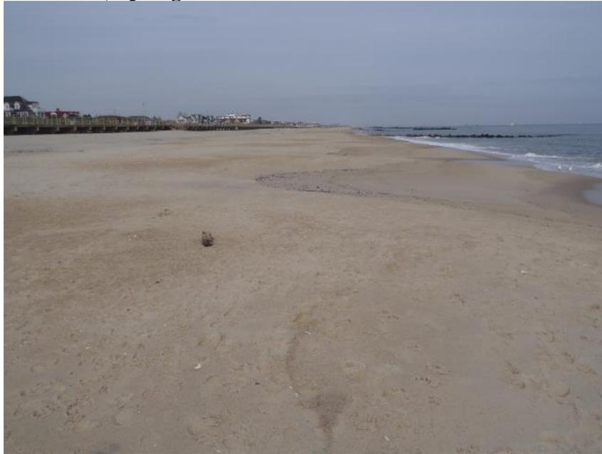
The dune is slightly lower and narrower at Mercer Avenue with a distinct separation from the boardwalk. The storm barrier was not built at the time of the fall 2018 survey. The beachface slope ending in 4 feet of water begins at the seaward toe of the barrier. Offshore a substantial bar system exists.
