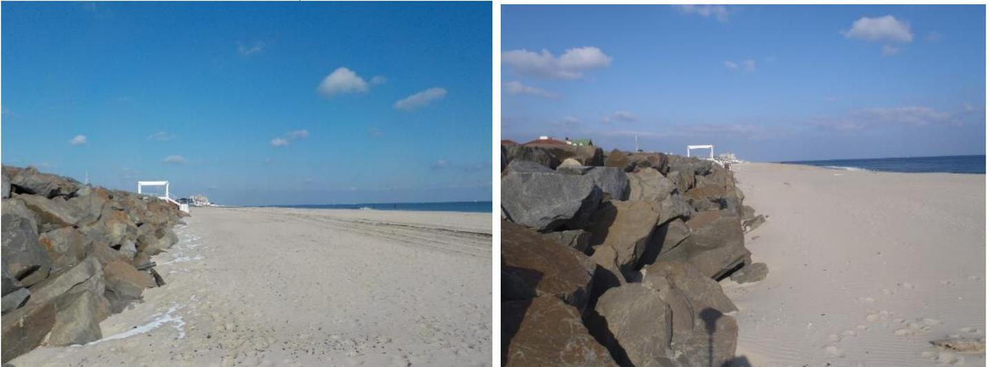
By December 11, 2017 (left), the project was complete and the beach had adjusted to the configuration shown below in the plots. The berm at elevation 10.0 remained close to the May 2017 position, but large changes took place offshore.
