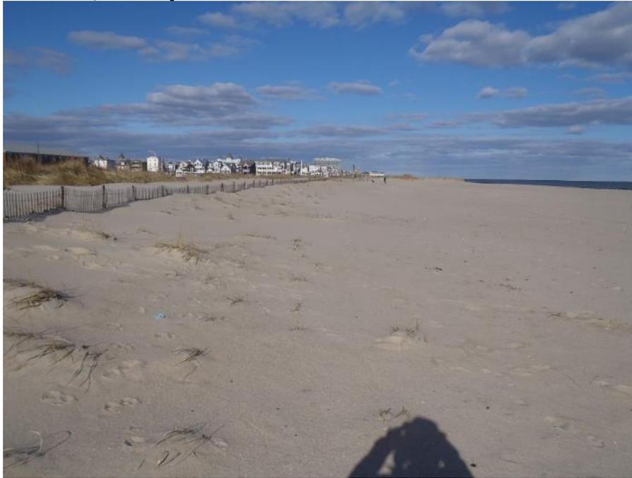
There is a dune between the boardwalk and the beachfront with about 200 feet of dry beach seaward at the USACE design elevation. There is a terrace offshore with a bar present as of November 2018.
