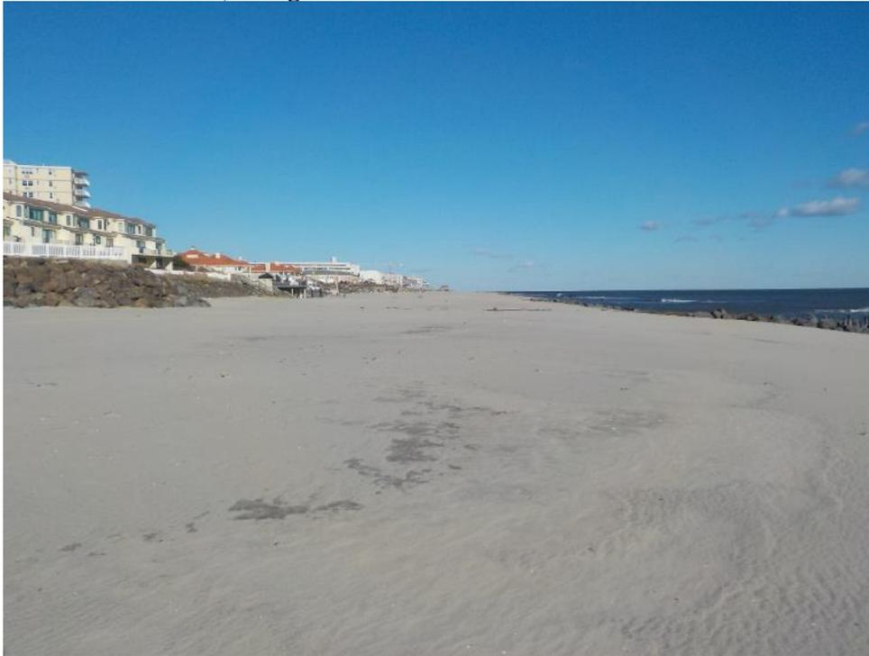
Located in the northern limit for the Phase III USACE beach restoration project, this location starts at a bulkhead, then extends across 250 feet of elevation 10.0 beach to the berm crest. The 10.0-foot elevation represents the project design elevation for the berm. Berm retreat did occur as sand moved offshore to start a bar system.
