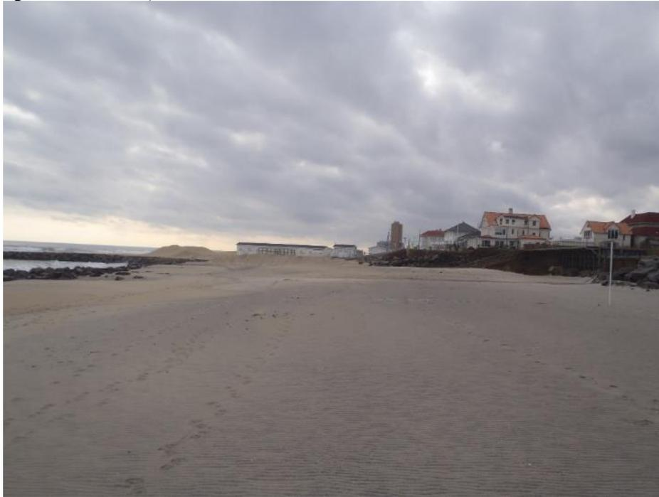
This is the southernmost site in Deal with the bluff protected by armor stone. The beach has retreated this year, post project with about 70 feet of the 10.0-foot elevation berm remaining. The beachface slopes seaward and intersects a low gradient terrace offshore.
