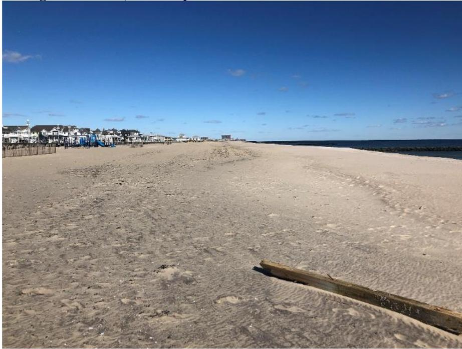
This new site is located approximately 300 ft. north of the Shark River Inlet north jetty. The elevation 10-ft berm extends seaward from the boardwalk by 180 feet. The 2017 offshore bar vanished in 2018, but the elevation of the surface decreased.
