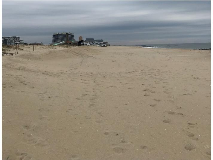
sand volume added during 2014 remains in place (Nov. 21, 2017) with minor variations leaving the berm virtually unchanged on November 30, 2018 (right). There was a storm ridge pushed up by Nov. 2018.
