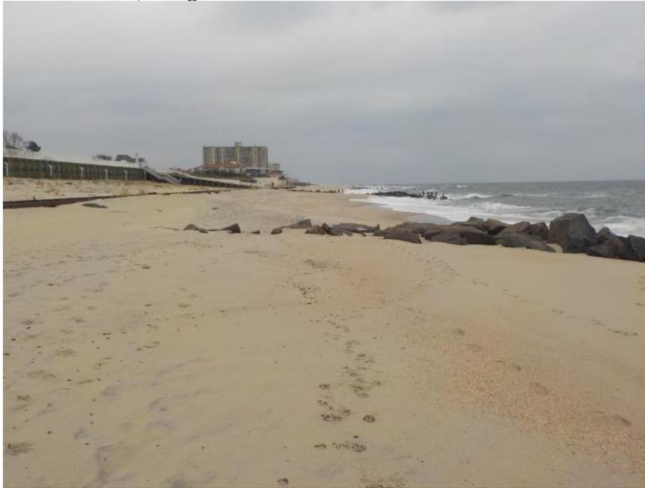
Located in the Elberon groin field, this location was completed during 2016 and clearly has adjusted with beach width reduction and sand deposited offshore in a very large bar system. The rocks above are now exposed.
