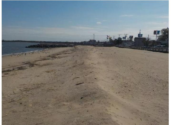
This site was moved to the public bathing beach in 2009. The photograph on the left shows the shoreline on September 20, 2017 with a small storm barrier pushed up onto the berm. A truck fill project in 2013 added 14,000 cu. yds. of sand. The photo on the right shows the beach width and berm on October 5, 2018, again with the ridge pushed up as of early-October.
