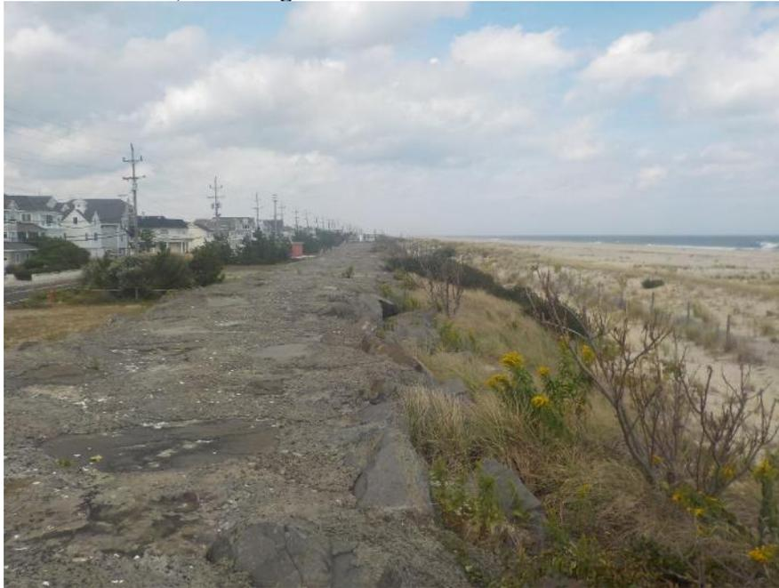
This site along the Sea Bright seawall shows the dune and wind deposited sand among the seaward facing rocks. The fence line showing in the photograph is the alignment that initiated sand deposition to create the dune system. Grasses propagate seaward across the dry beach because of the low pedestrian traffic and absence of any beach raking maintenance.
