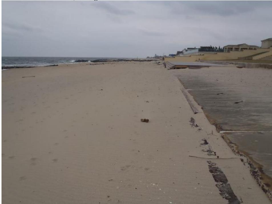
This location is also within the Elberon groin field. The beach is under 100 feet wide to the berm crest. The offshore terrace is 200 feet wide indicating considerable profile adjustment since 2016.
