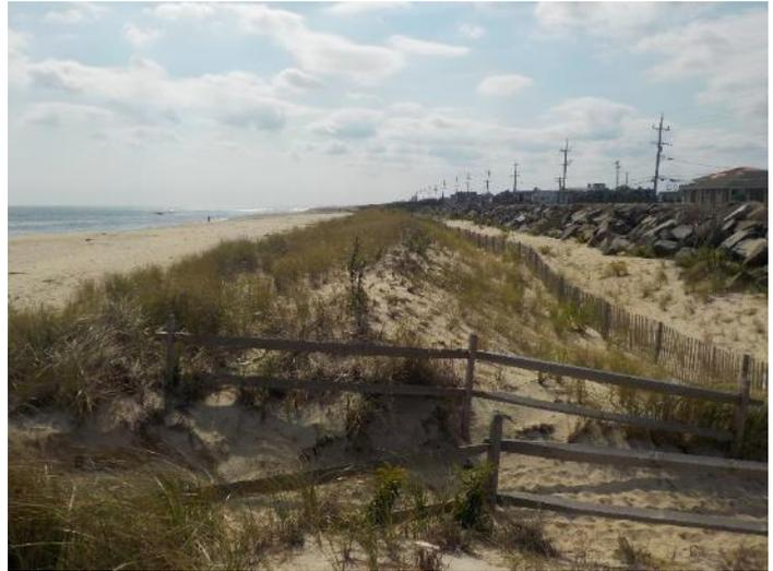
This site is near the northern limit of the initial Federal shore protection project. The left photo shows the seawall and the line of dunes looking south on Jan. 10, 2018, while the right photo (Oct. 1, 2018) shows a southerly view from the dune crest. This dune was not built as part of the project, but has developed as time passed around one line of fencing.
