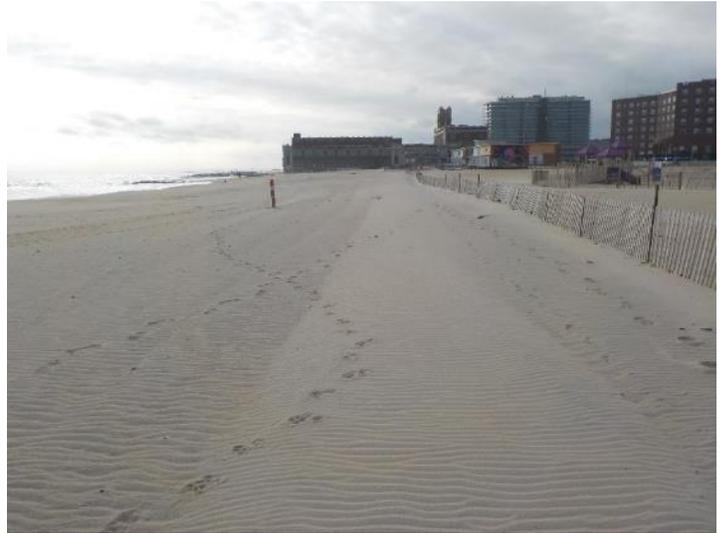
This site is the northernmost location in the Phase II part of the Monmouth County project. The left photo was taken Nov. 28, 2017 and shows the sand fence placed primarily to restrict access to the boardwalk reconstruction. Sand did accumulate at the toe of the fence as the boardwalk work continued. No storm ridge was pushed up as of mid-December 2018.
