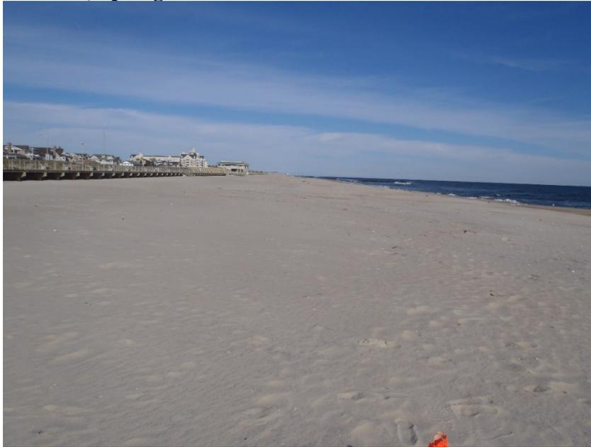
This site has a narrow dune with the boardwalk seaward of it without the storm barrier sand ridge (as of Nov. 14<sup>th</sup>). There is a 100-foot wide, 10.0-foot elevation beach seaward of the boardwalk with a significant offshore bar system present.
