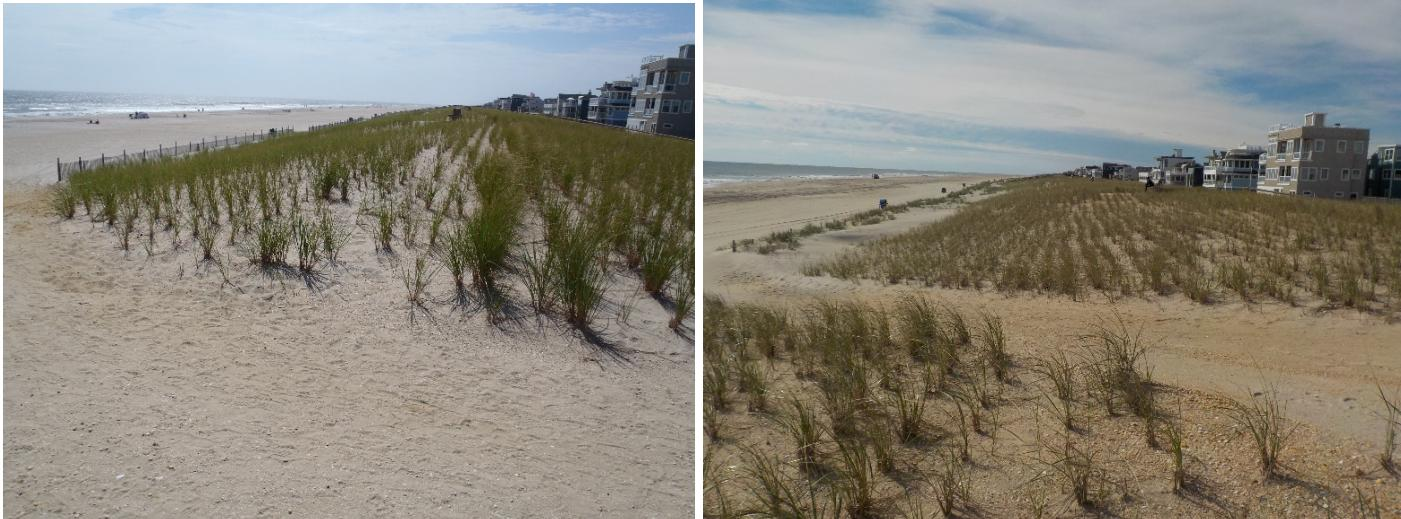
The photos show the view to the south from the dune crest at the 81<sup>st</sup> Street location (left photo taken September 14, 2017 and right taken October 16, 2018). The right photo shows sand that accumulated landward of the dune fencing. This is displayed in the cross section below.
