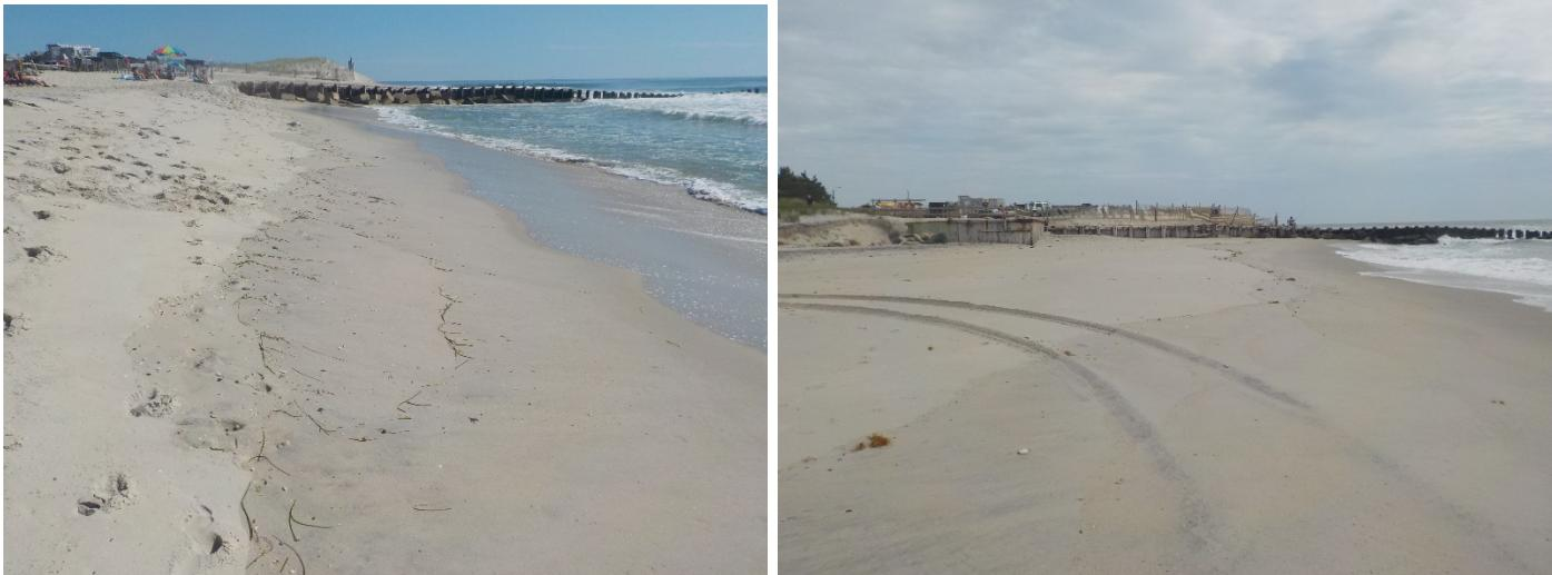
The Holgate entrance profile lies immediately downdrift of the Holgate terminal groin and the photos show the changes at the seaward portion of the berm (left photo taken September 13, 2017 and right taken September 17, 2018). By September 2018, the bulkhead at the edge of the municipal parking lot was exposed to wave activity. Also of note is the loss of the engineered dune on the north side of the groin, indicating the structure's inability to hold the beach fill design template.
