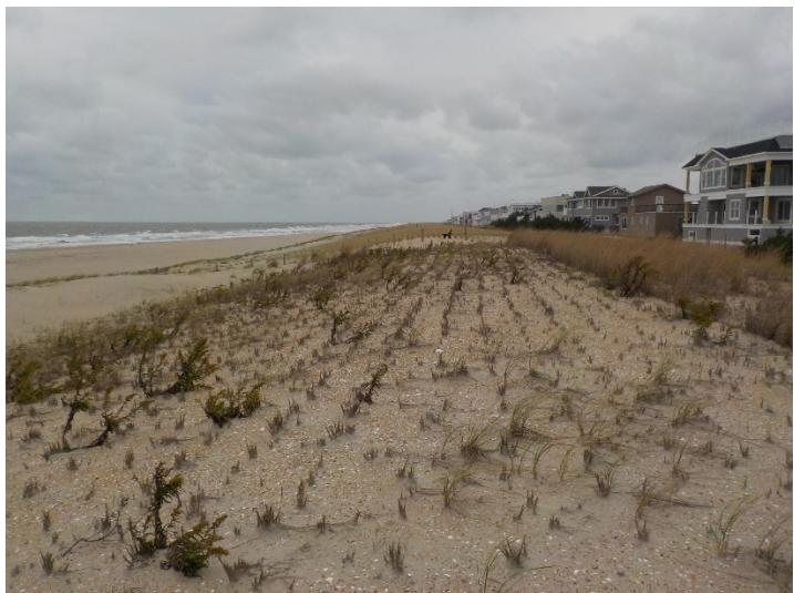
View to the south from the dune crest at the Tranquility Drive location (left taken September 15, 2017 and right taken November 9, 2018). The engineered dune remained in position with the seaward edge gaining in elevation as the result of wind-blown sand that was trapped by dune fencing.
