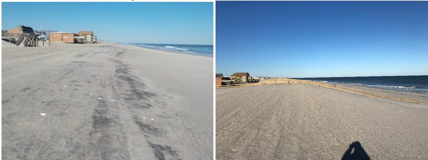
The left photo taken October 31, 2017 shows the berm as a result of the state/local “betterment” that occurred in May 2017 (after the CRC spring 2017 survey). The right photo (taken December 18, 2018) was taken from the crest of the new engineered dune located over 100 feet seaward of the fall 2017 dune. The beachfill was completed at this location by November 2018.
