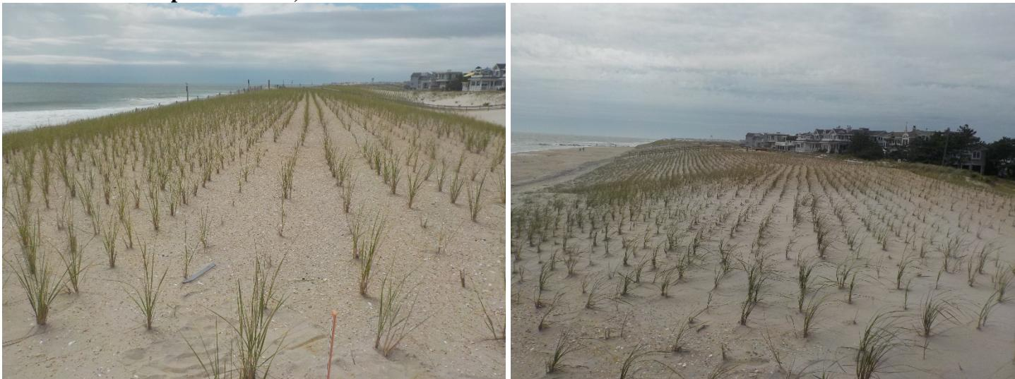
The photos at the Dolphin Avenue profile show the alteration of the landward portion of the engineered dune (left taken September 13, 2017 and right taken September 17, 2018). In 2018, the crest was shifted landward to accommodate changes to the USACE dune template. The area was filled with sand and replanted to meet the elevation of the pre-existing dune. The right photo shows a new accumulation of sediment on the dune crest where windblown sand was trapped by vegetation.
