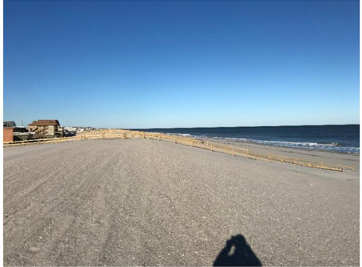
The left photo taken October 31, 2017 shows the berm as a result of the state/local “betterment” that occurred in May 2017 (after the CRC spring 2017 survey). The right photo (taken December 18, 2018) was taken from the crest of the new engineered dune located over 100 feet seaward of the fall 2017 dune. The beachfill was completed at this location by November 2018.
