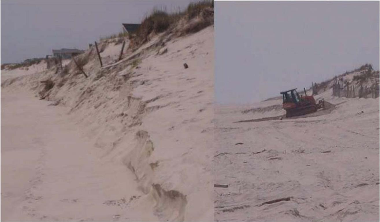
Photograph taken May 2, 2005 following erosion of the seaward dune slope during late winter northeast storms. This damage to the dunes was repaired all along the Long Beach Island shoreline using a bulldozer to harvest sand returning to the beach during the following weeks of calm sea conditions.
