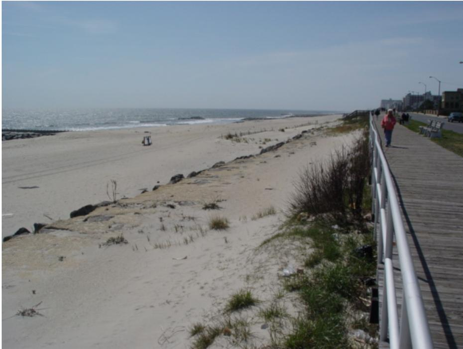
Figure 50. April 12, 2006 view to the south showing the beach fronting the rock revetment built in the 1960's to protect the bluff from erosion that had breached prior bulkhead structures. This wall occupies the original location of the boardwalk built over the beach at that time.
