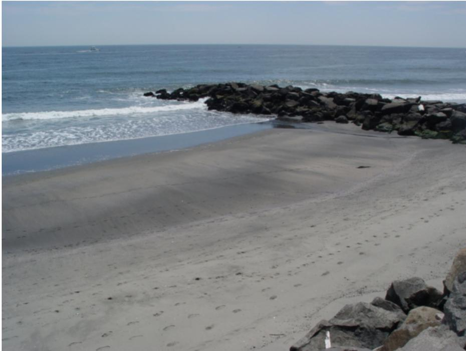
Figure 59. This June 21, 2006 view of the Roosevelt Avenue beach shows an unusual situation where sand had built up to the point where a terrace extended half way out to the groin tip. The plots show a wedge of sand up to 5 feet above the zero elevation line. Loss followed during the next two surveys with some recovery seen following the final survey (#35).
