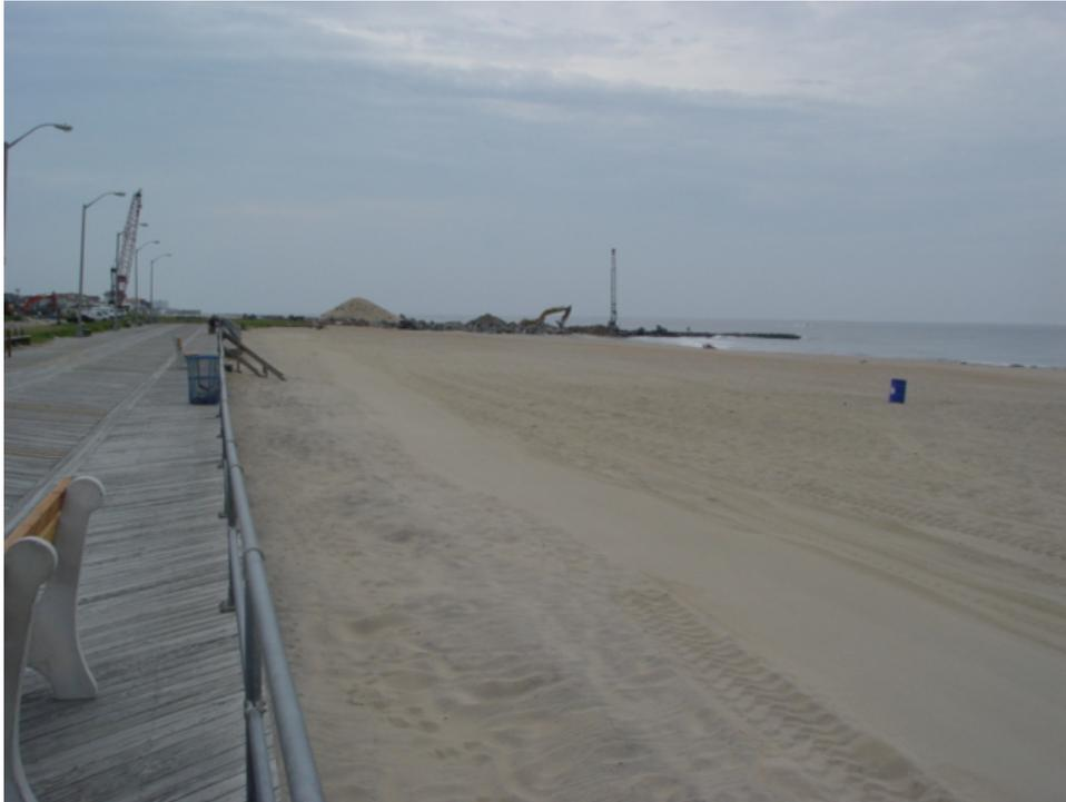
Figure 69. This view of the northern Asbury Park beach was taken June 20, 2006 and shows the terminal groin with the cranes on it rebuilding the Deal Lake outlet. The beach width has maintained a relatively constant value, which corresponds with the very slow rate that the Allenhurst beach grew due to limited sand by-passing of the groin.
