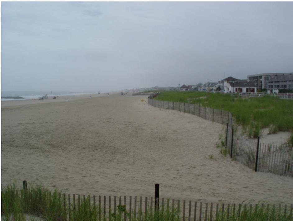
Figure 77. Dunes were incorporated into the beach project in Bradley Beach creating a totally new look for the oceanfront. The high tide came under the boardwalk in 1992 damaging most of it. The boardwalk was removed from the beach and rebuilt as a promenade on the seaward edge of the bluff. The western half of the dune field occupies the former position of the boardwalk. This photograph was taken June 26, 2006.
