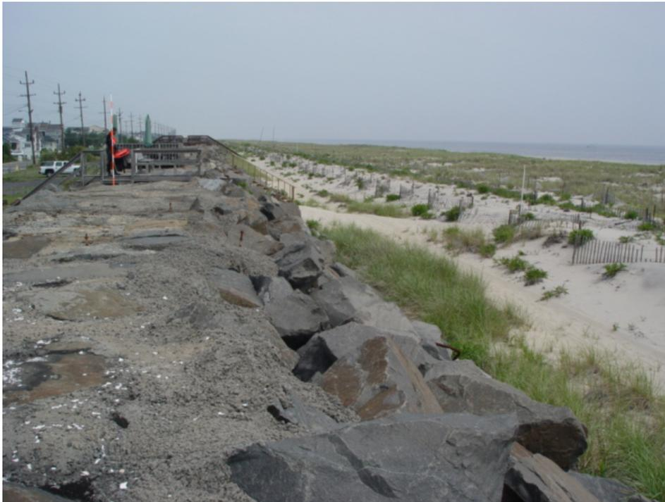
Figure 23. June 14, 2006 shows a view across the vegetated plain that is the back beach of this location. It is 440 feet to the zero elevation position from the seaward base of the seawall.
