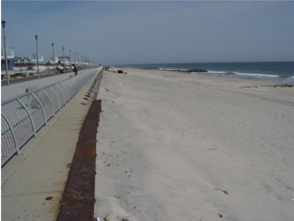
Figure 47. April 12, 2006 shows a view to the north along the Long Branch steel bulkhead built to protect the upland bluff decades ago. The wind transport has moved sand up to the top edge of the structure in places.
