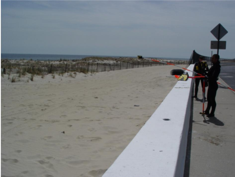
Figure 41. April 17, 2006 photograph shows a view to the south from Ocean Avenue. The bare area is an access zone to the beach. The dune is relatively modest in height, but the extra width of the beach provides substantial protection.
