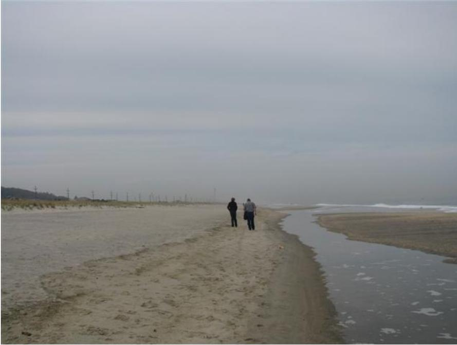
Photo taken November 4, 2008.. View to the north. Remember that prior to the 1996 fill at this site, the beach walkers in the picture would have been swimming in 16 to 20 feet of water 350 feet east of the seawall.
