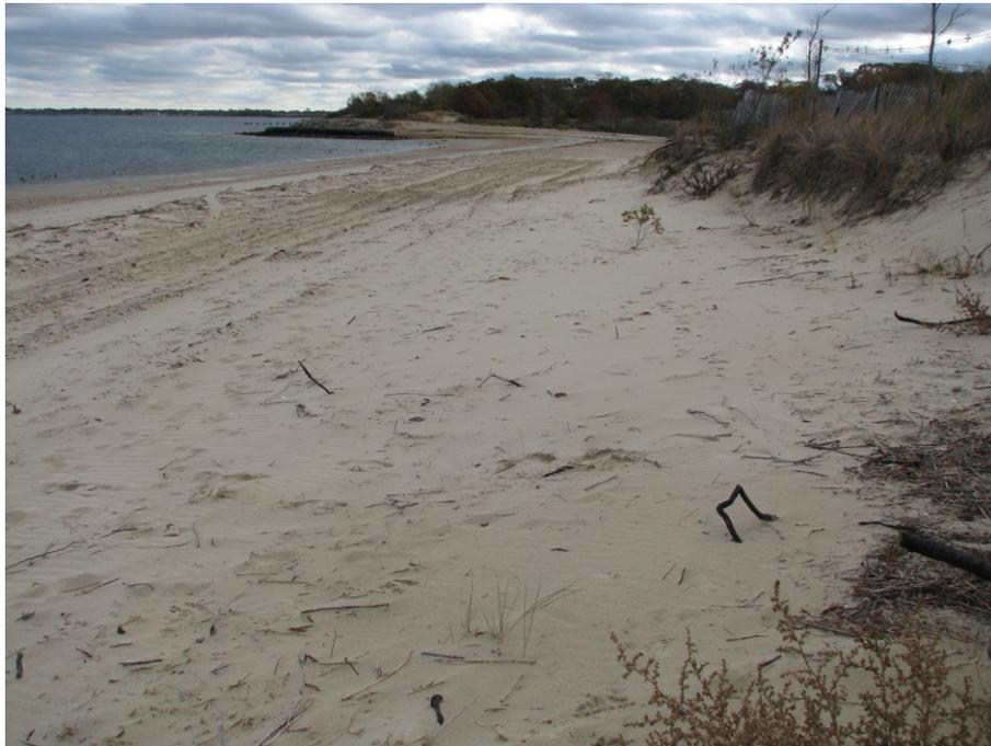
Comparing the profiles over the year, the profile location lost volume (-2.16 cu yd/ft) and the shoreline moved landward (-14.77 ft). Raritan Bay northeast storm waves cut into the dunes and pushed back the beach.
